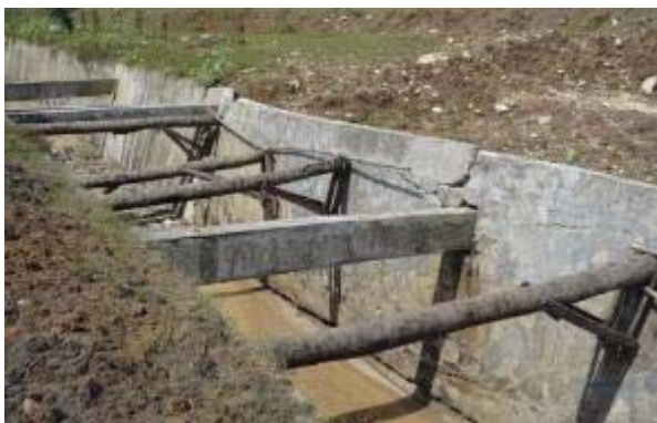
Figure 3.5.6: Damaged Drain Ditch cause by Expanded Soil in Indonesia
