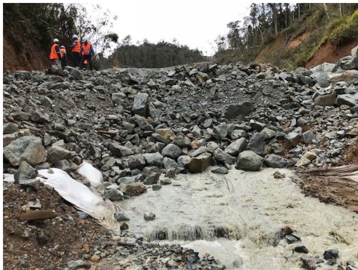
Photograph 4.6 Underdrain cover by 5m thick NAF (non-acid forming)
