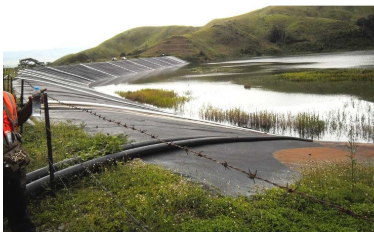
Photograph 4.4 Tailings dam in Kainantu Mine
