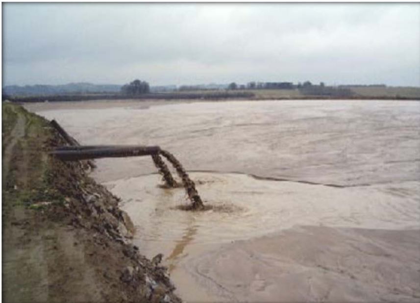
Photo 1: Tailings discharge into a dam
