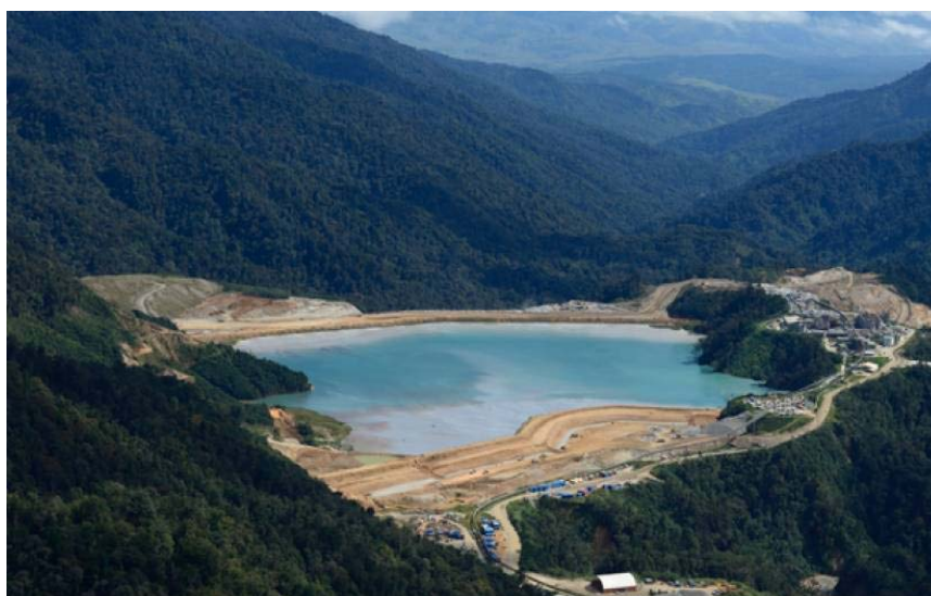
Photograph 4.5 Hamata tailings dam (Saddle dam in front, Main dam in the back)
