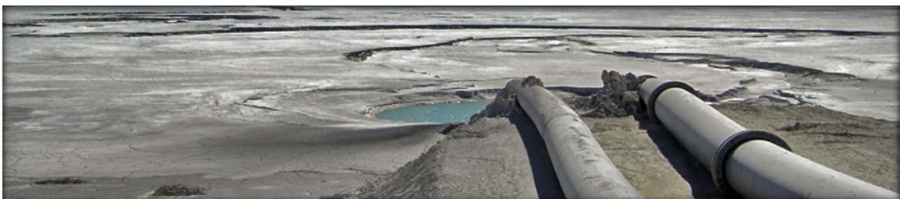
Photo 6: Tailings Pipeline Facilities
