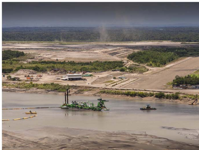
Photograph 4.3 Dredging in Ok Tedi River and East Bank dumping area
