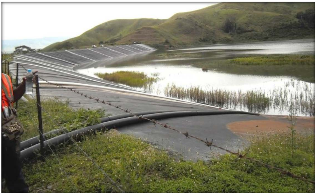
Photo 8: Tailings Dam in Kainantu Mine, Eastern Highlands Province
