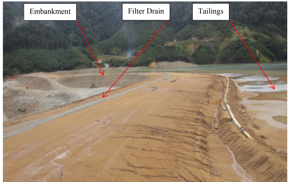
Photo 2: Upstream method used at Hidden Valley Mine, Morobe Province
