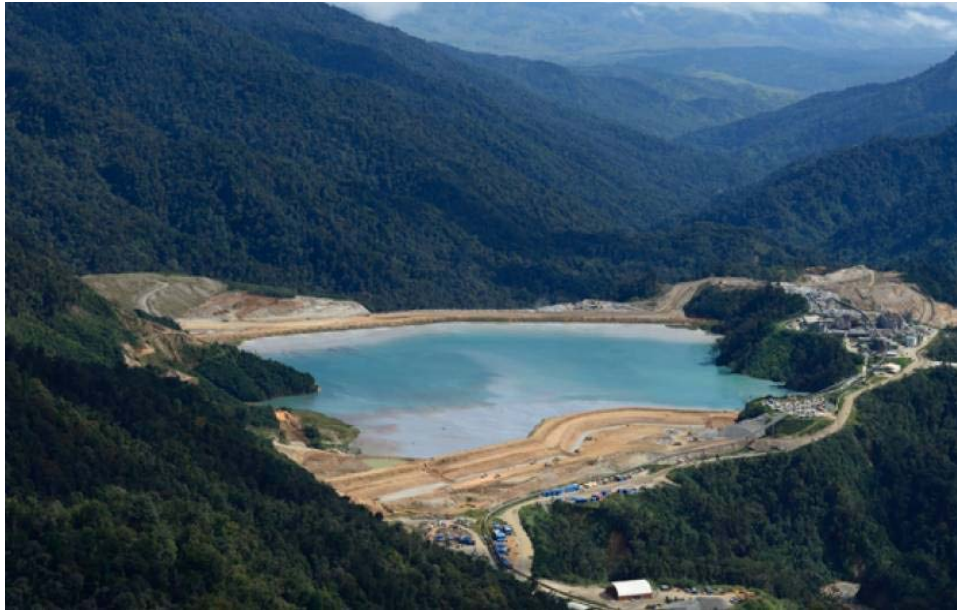
Fig.1 Hamata tailings dam (Saddle dam in front, Main dam in the back)
