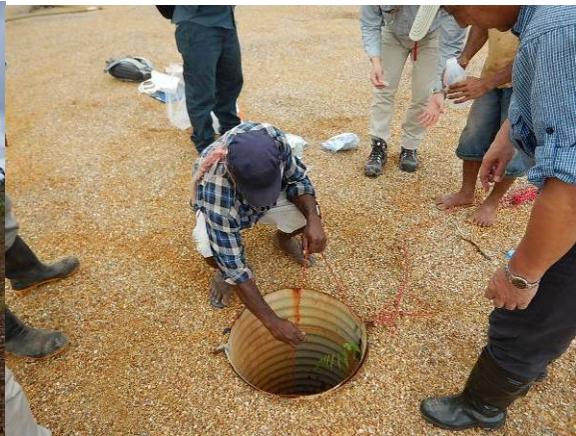
Photo 2: Pumping well of leachate in Vat E
