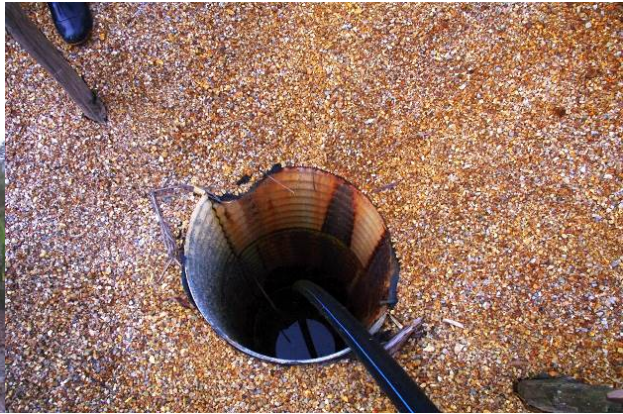
Photo. 2 Pumping well of pregnant solution
