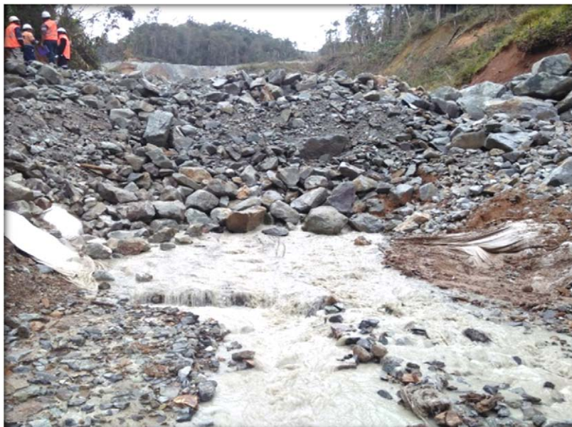
Photo 7: Waste Dump Underdrainage at Hidden Valley Mine, Morobe Province.
