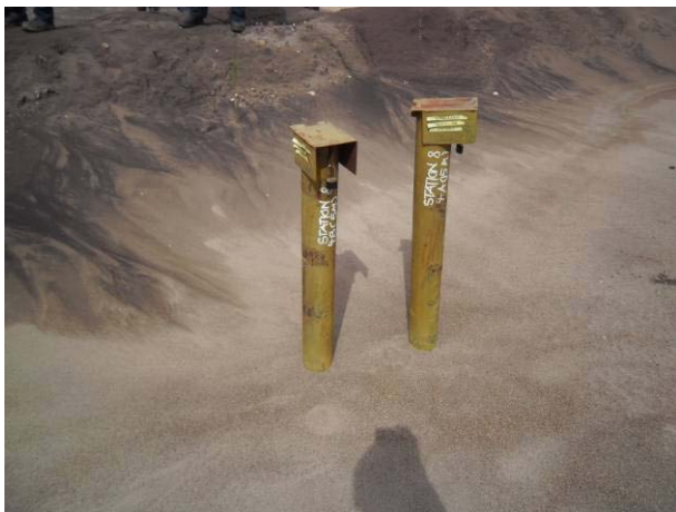
Monitoring wells installed at the Bige stockpile
