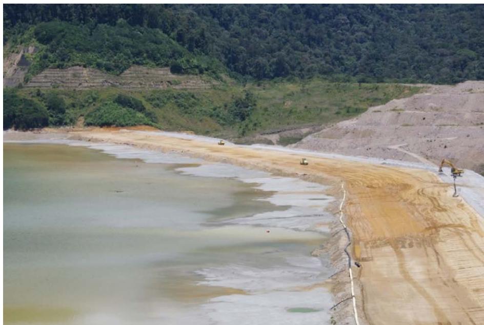
Fig. 3 Construction for heightening of embankment of Main dam
