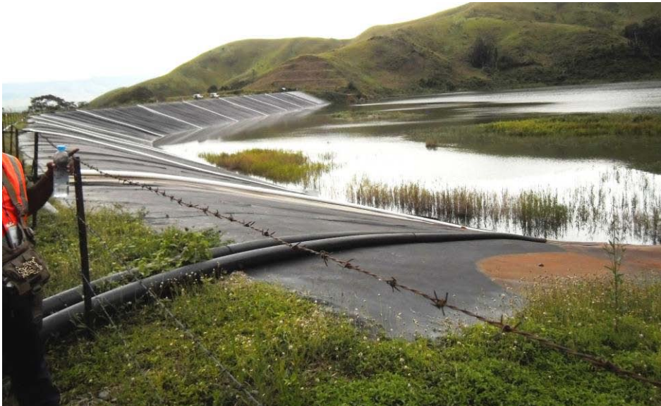
Fig. 3 Current Tailings dam in Kainantu Mine
