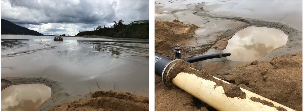
Fig.3 Discharging of tailings at the Saddle dam
