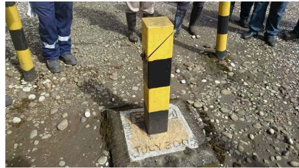
Monitoring wells installed at the Kiunga operation center
