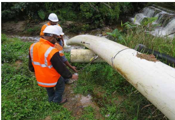
Photo 10: Water sampling at a discharge point
