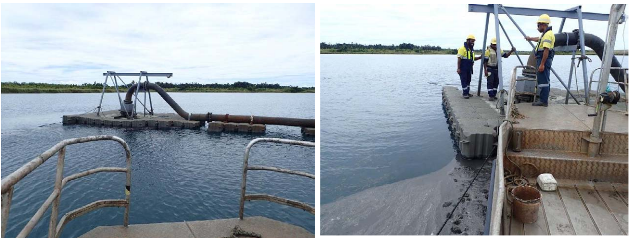
Fig. 2 Deposition of pyrite concentrate in Pit-3 at Bige
