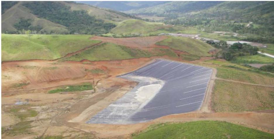
Fig. 2 Tailings dam in Kainantu Mine under construction
