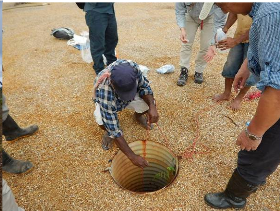
Photo 2: Pumping well of leachate in Vat E
