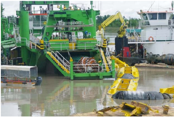
Dredger at Bige
