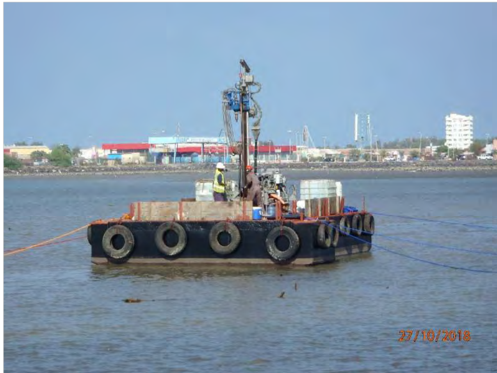
Photography 1: Floating pontoon
