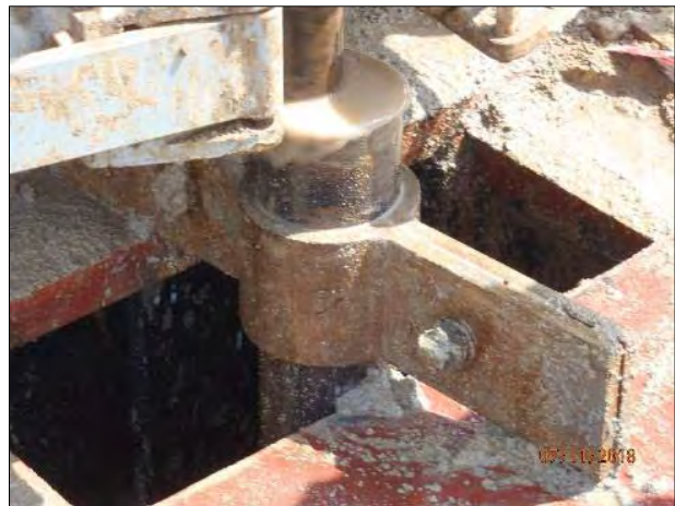
Photography 15: Restoration of carotage with adjuvant in traffic waters
