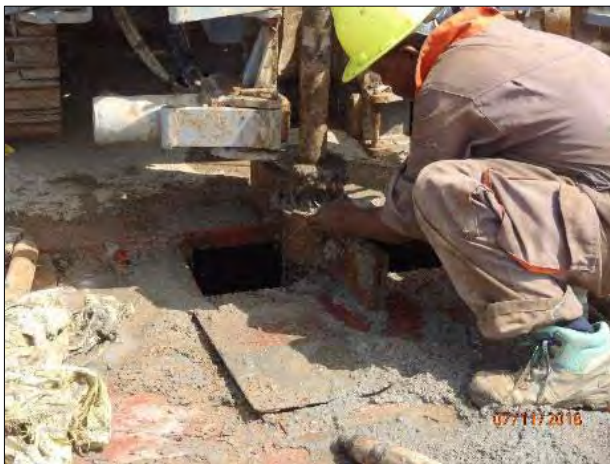
Photography 16: Sediments out of tubing during carotage
