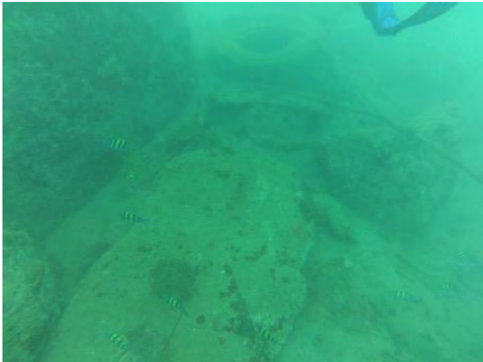
Photo 7: Structure of the two dolphins in Tadjourah port (underwater photos)
