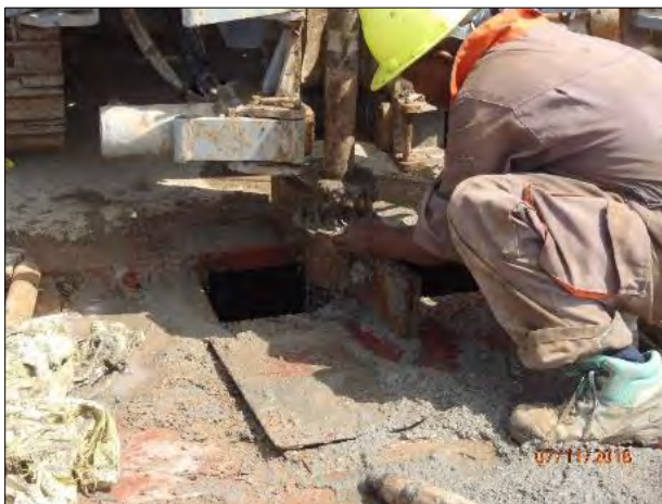
Photography 16: Sediments out of tubing during carotage
