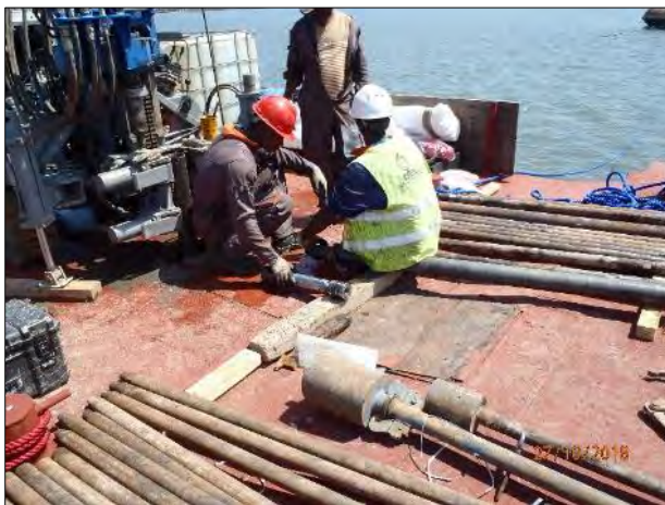
Photography 18 : Recovery of samples in the carrot
