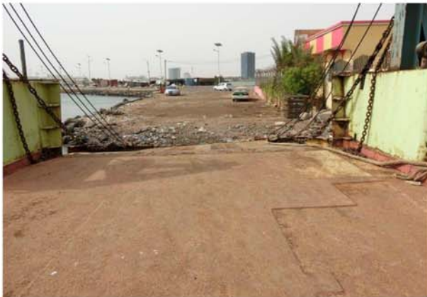
New Ferry Terminal Area at Djibouti Port View from sea side to land side (2 nd July 2018)
