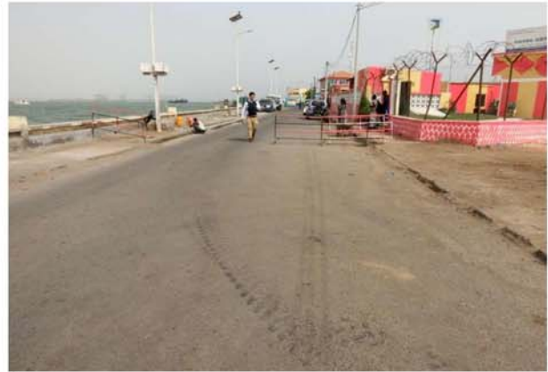
New Ferry Terminal Area at Djibouti Port View from entrance to Coast Guard (2 nd July 2018)
