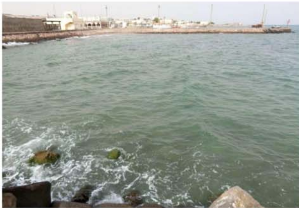
New Ferry Terminal Area at Tadjourah Port View new reclamation area for new terminal and present ferry terminal (4 th July 2018)
