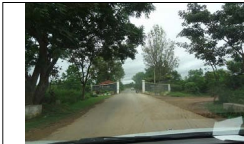
Photo 3-46 Airport Access Road (1)
