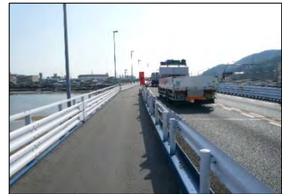
Photo 2-2-3 Example of Bridge Pavement
