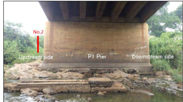
Photo 2-2-1 Current Condition near the Bridge Pier
