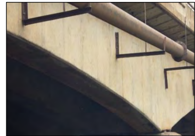
Photo 2-2-4 Water Pipes of the Existing Bridge
