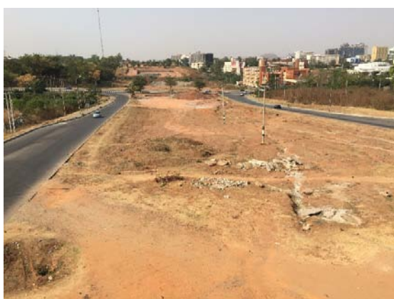
Extension of expressway
