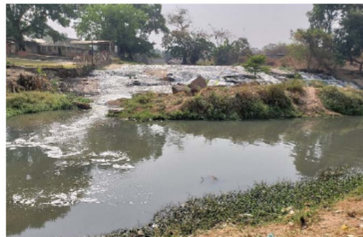
Leak of sewage water into river in FCC
