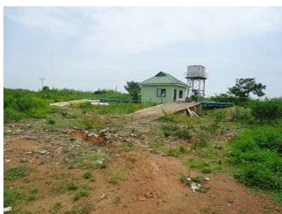
Weigh Bridge (under construction)
