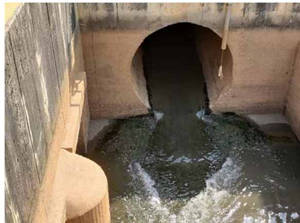
No.2 Inflow of Wastewater at Wupa Basin Sewage Treatment Plant
