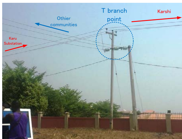
Photo 8.1.1 Typical T Branch for Power Distribution to Various Communities
