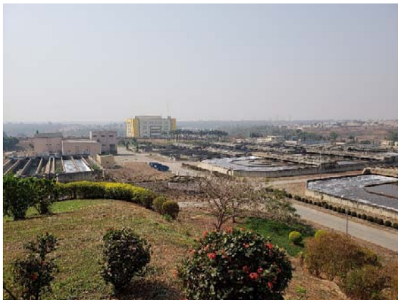
No.1 Wupa Basin Sewage Treatment Plant
