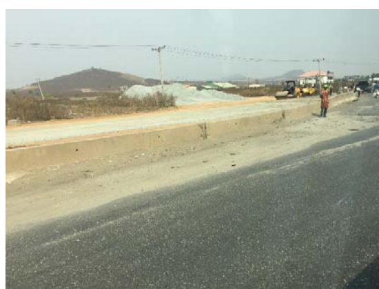
Widening of highway
