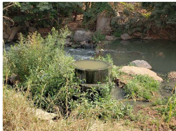
No.2 Overflow of Wastewater from the existing Manhole
