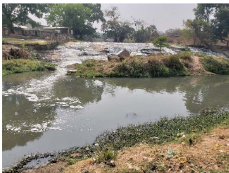
Leak of sewage water into river in FCC
