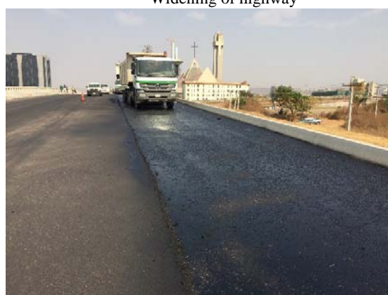
New construction of flyover section in the CBD
