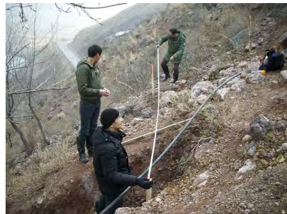
Picture 2-4 Installation of Monitoring Pole for Landslide
