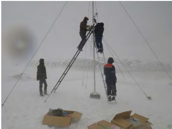
Picture 2-9 Installation of Meteorological Observation Equipment
