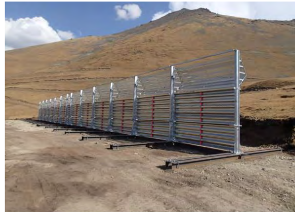
Picture 2-10 Pilot Project (Construction of Snow Fence)
