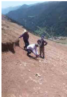
Ground Topographic Survey (Slope)
