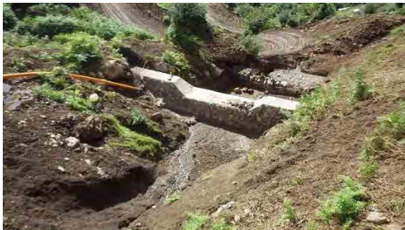
Masonry high wall
