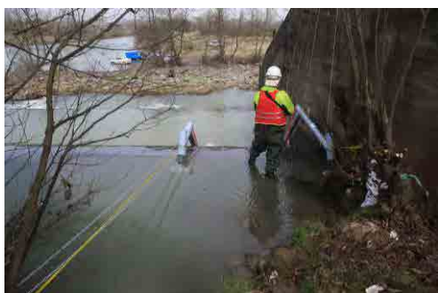
Fishway installation on Pasikhan Dam on 9 Mar 2018
