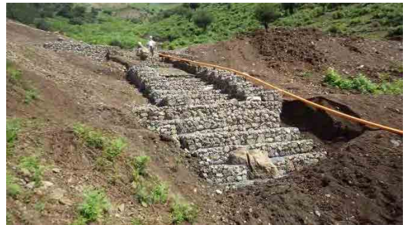
Stream bed protection under the wall of 2017
