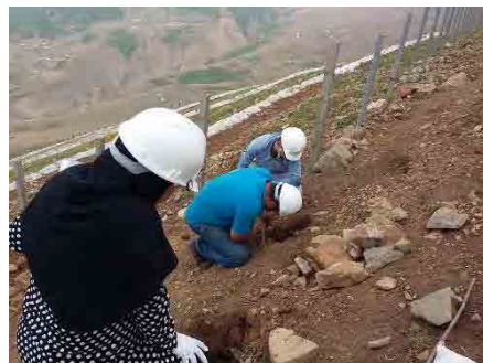
Progress inspection of post of fence
