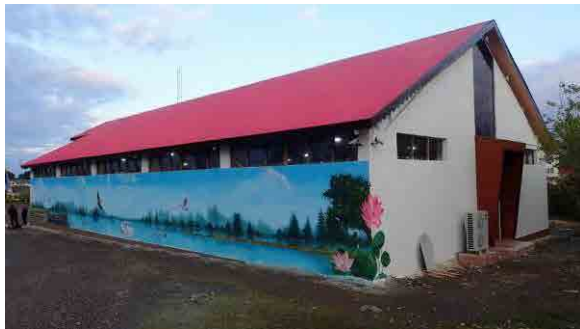
Exterior of the building (back side)
