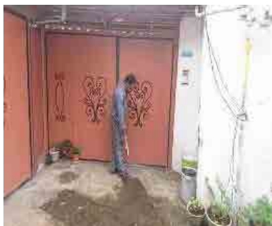
One of the completed house connection work
