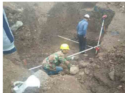
Progress inspection of excavation work
