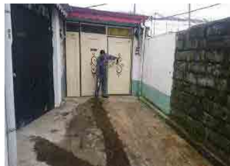
One of the completed house connection work
