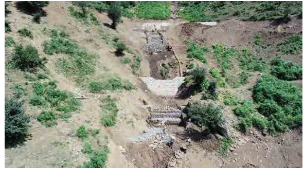
Construction under JPA 2017
