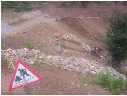
Signboard for safety
