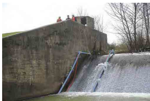
Fishway installation on Pasikhan Dam on 9 Mar 2018
