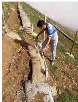
Progress inspection of the terracing in the slope area
