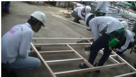
[Practical training photo: carpentry course]
