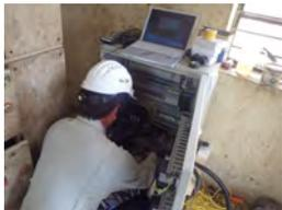
Connecting wires to control panel
