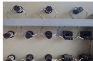
Modification of existing control panel (removed contact)
