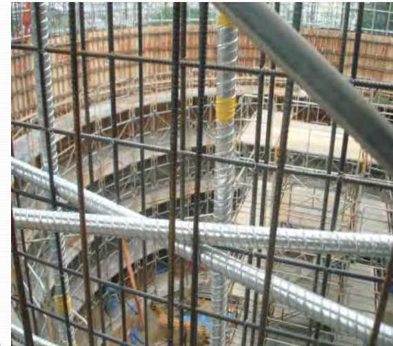
Close up; Tendon Arrangement at the Pilaster Galvanized sheaths are clearly shown here.
