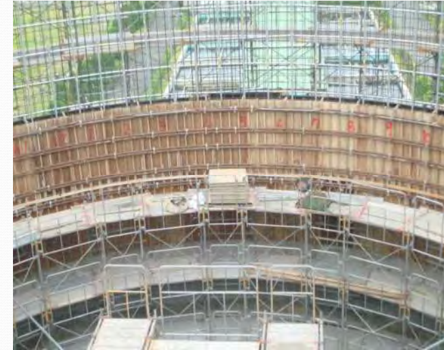
Form Work+ Arrangement of (Vertical Pre stressing bars+ Horizontal Pre-stressing Strands )
