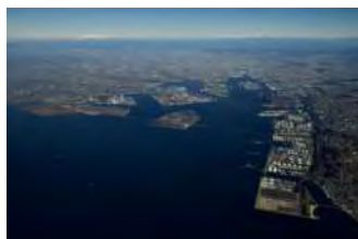
Overview from south
