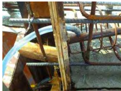
Grouting Tube Arrangement at the Site
