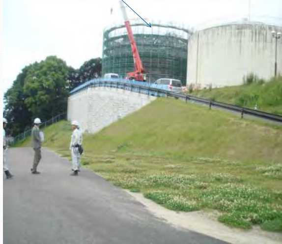
The Structure under Construction
