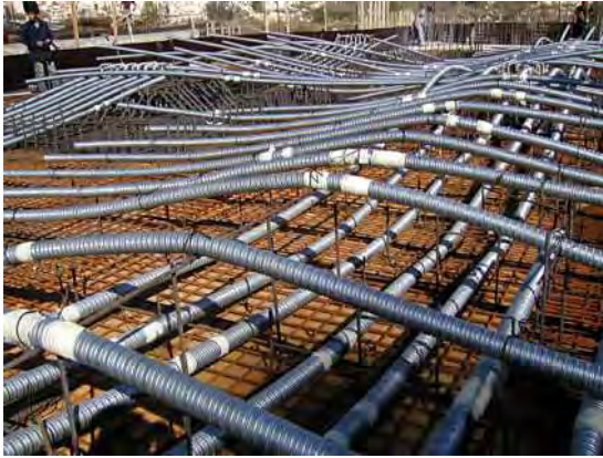
Bonded Post tensioning System
