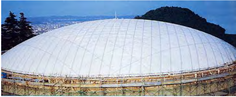
Blowing up of membrane - under construction
