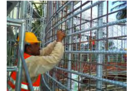
Sheath Arrangement in a PC Tank
