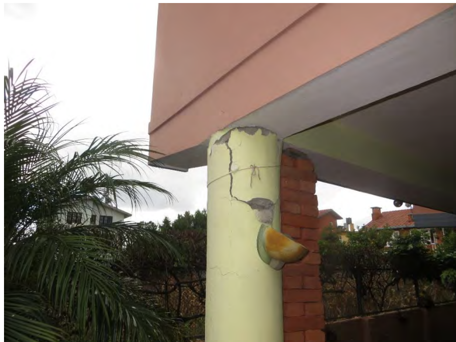
Figure 7. Crack in columns of ground floor due to Gorkha earthquake
