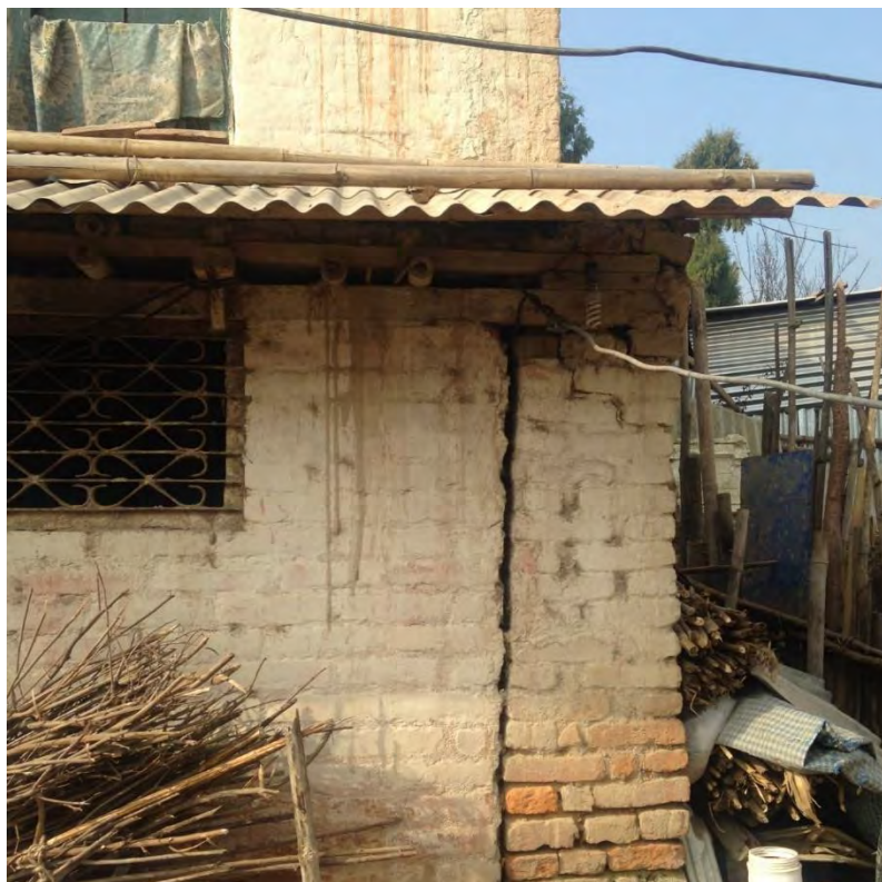
Figure 2. Crack formed in the corner due to Gorkha earthquake
