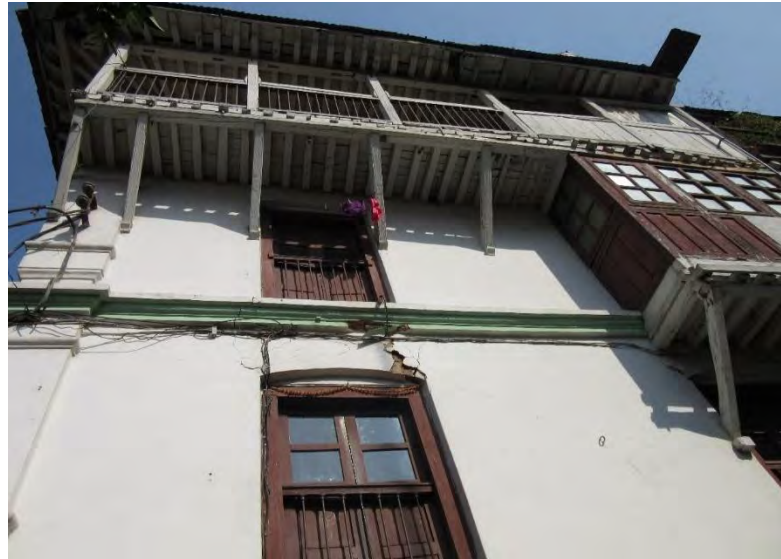
Figure 4. Crack above the window due to Gorkha earthquake
