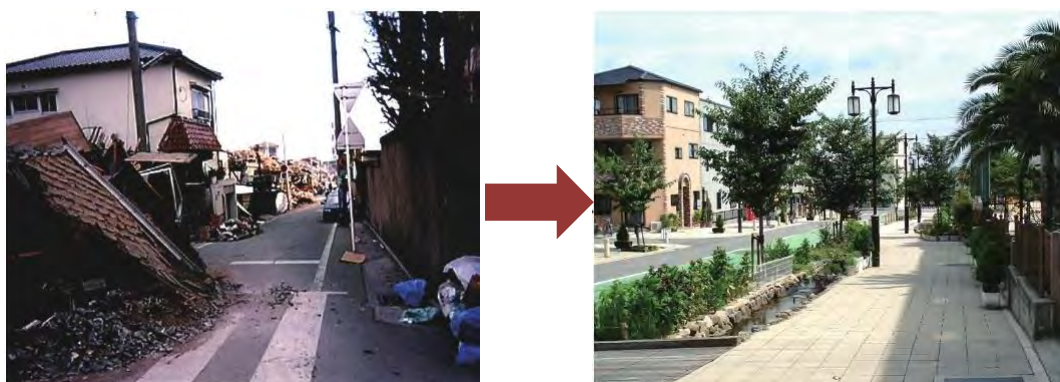
Figure 2-2 Image of Build Back Better (The safety of the town was improved after rebuilding roads as wider ones (Same location in Kobe city))
