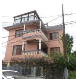
d) RC non-engineered (soft story)
