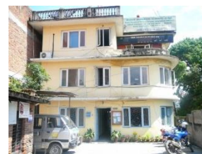
c) Brick masonry with cement mortar
