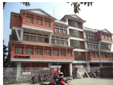
b) Municipality building
