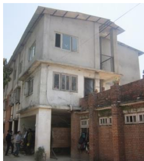
a) School: Brick masonry with cement mortar
