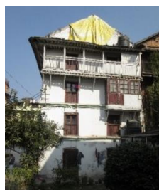
B) Brick masonry with mud mortar
