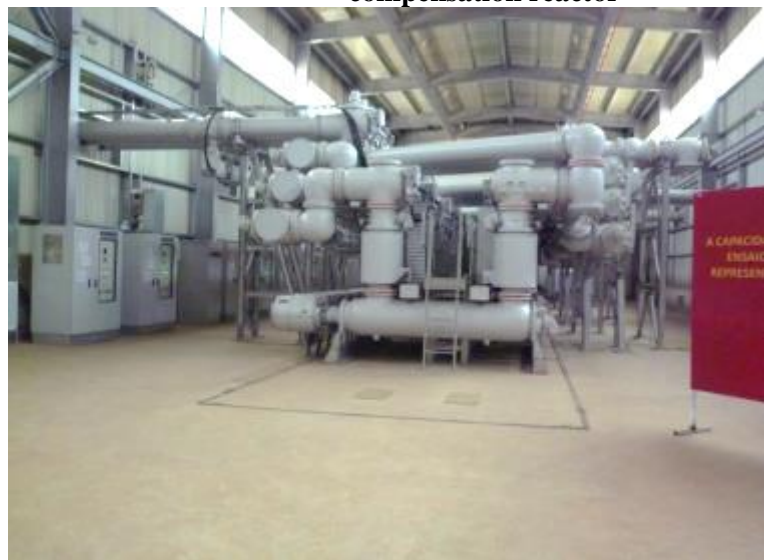
Figure 7-17 Indoor type gas-insulated switchgear
