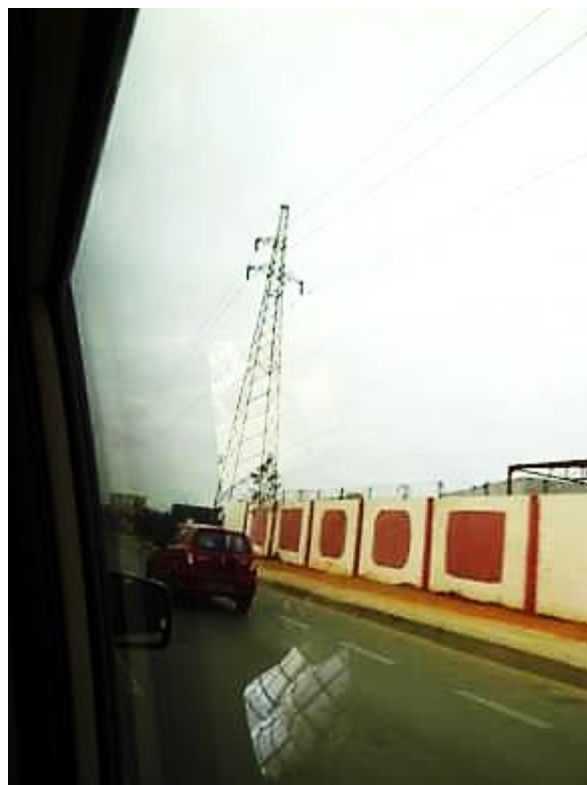
Figure 7-6 66 kV one circuit angle tower
