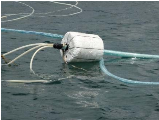
3 airline tubes from compressor used by the divers inserted to the plastic hose with styro bouy to inject air to the HDPE ring.
