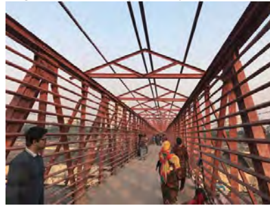
Image 9: Foot over bridge across platform
