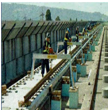
Rail installation by portal cranes
