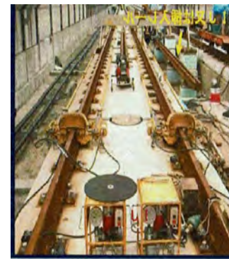
Rail Setting and installation of insulation joint
