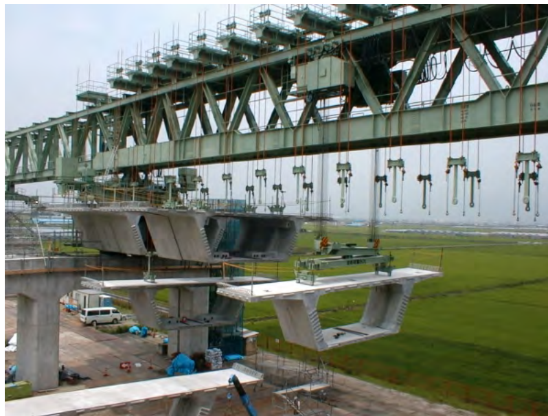
Figure 4.5.37 The Span by Span Method Girder Erection
