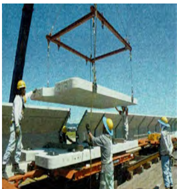
Lifting up concrete slab and loading onto the trolley
