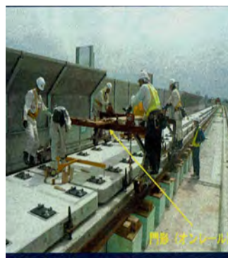
Laying the concrete slab
