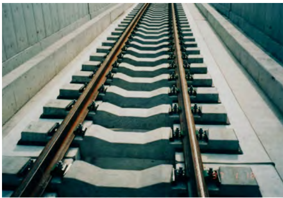
Non-Ballast Concrete Bed with PC Sleeper embedded in half of the Rubber Box
