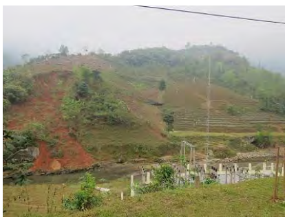
Photo 2.5 Status of the unstable slope close to the power generation facility (Lao Cai Province)
