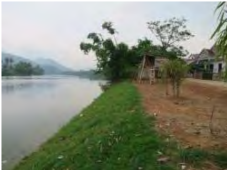
View of repair of a riverbank slope on a tributary of the Gianh River in Quang Binh Province (work completed in September 2014)
