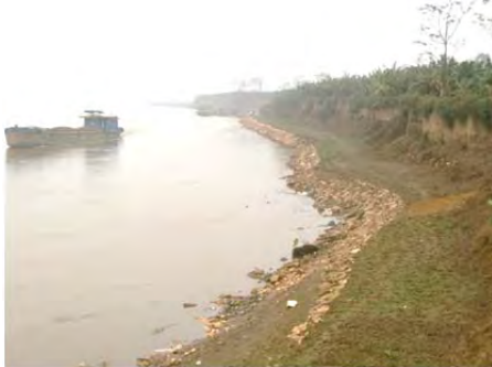
Photo 4.5 Riverbank protection major method by stacking stones seen in Vietnam (Left: Stacking stone only, Right: Stacking stones between concrete frame)
