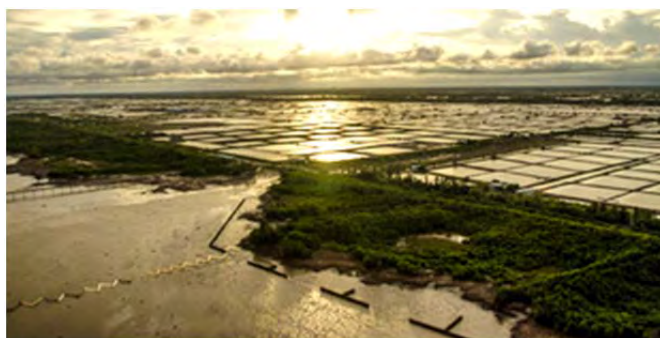
Photo 5.1 T-shaped breakwater on the Mekong Delta coast by GIZ
