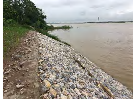
Photo 4.5 Riverbank protection major method by stacking stones seen in Vietnam (Left: Stacking stone only, Right: Stacking stones between concrete frame)
