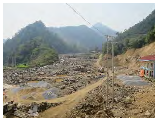
Photo 2.8 Damage situation at Nam Pam commune (Son La Province) Several slope failures are found in the upstream part. Flash floods deposited soil and rocks in the valley with a width of 30m to 100m. (Taken by the survey team, March 2018)
