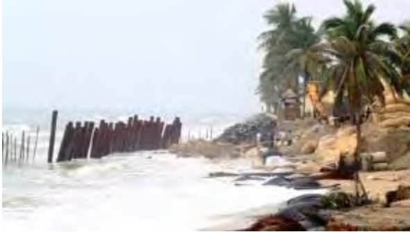
Photo 2.11 View of coastal erosion damage in Quang Nam Province
