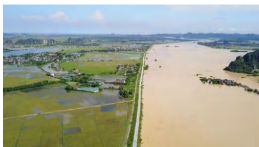
Water level reached the near dike top Hoang Long River (Ninh Binh province)
