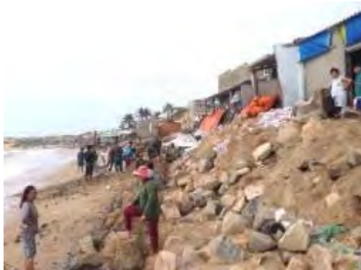
Photo 2.12 View of coastal erosion damage in Binh Thuan Province
