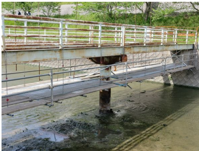
For example of Scaffold
