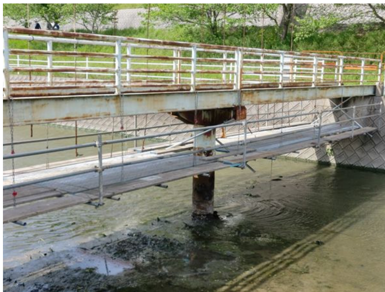
For example of Scaffold
