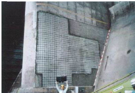
Cleaning of Concrete and Rebar
