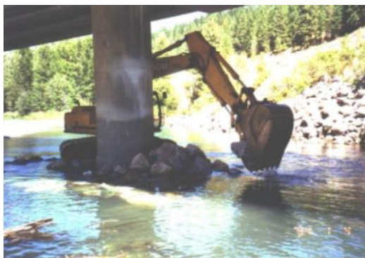
Placing Special Heavy Loose Rip Rap
