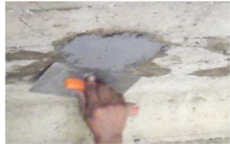
Filling up in Patching
