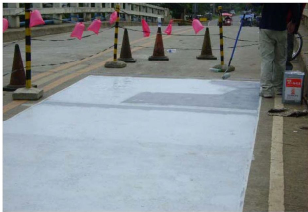
Photo 17-1 Rubberized Membrane Method
