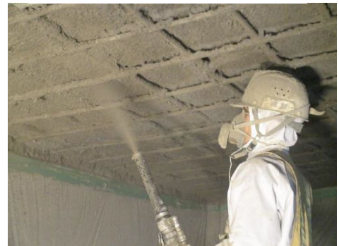
Spraying repair mortar
