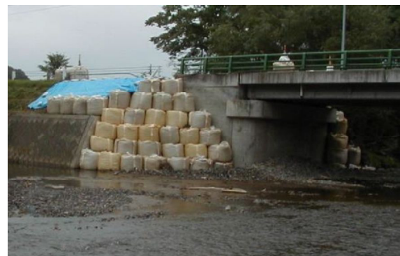
Photo 3-14-4 Placing Sand Bags
