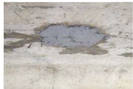
Curing after Patching
