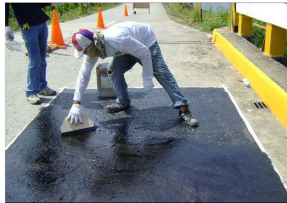
Photo 17-2 Asphalt Compound Method
