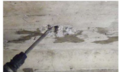
Removal of defect concrete
