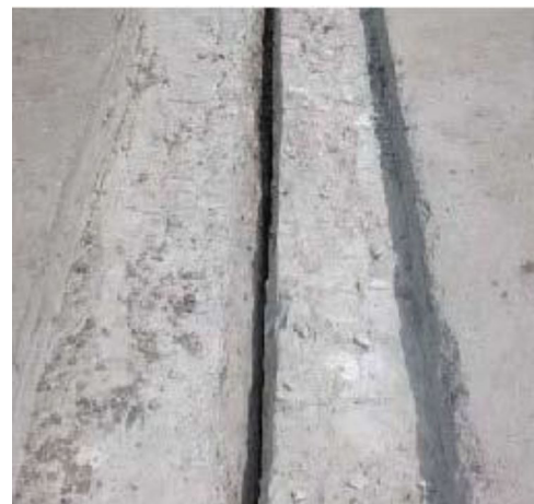
After removing Sealant of Asphaltic plug joint
