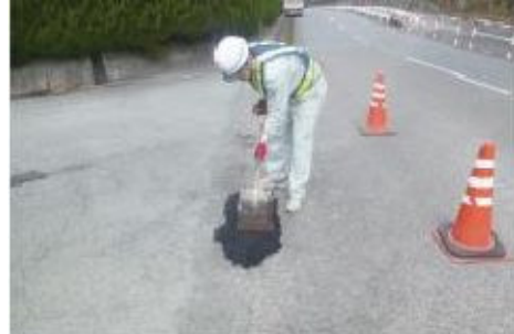
Photo5-3 Patching of Repair Material
