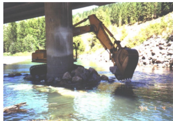
Placing Special Heavy Loose Rip Rap
