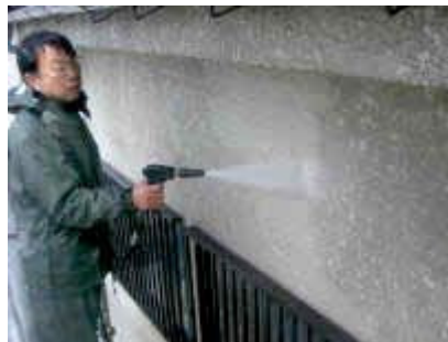
Fig.2-13 Cleaning concrete surface by jet water
