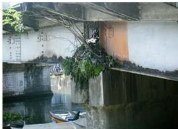
Photo 1-1-3 Vegetation in deck / girder
