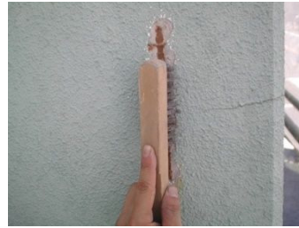
Fig.2-23 exposed Rebars (small area) Fig.2-24 Treatment of exposed rebar by brush
