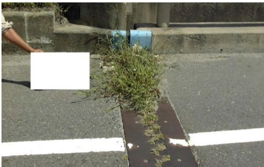
Fig.2-7 Blocked expansion joint
