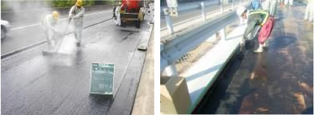
Figure 4-17 Waterproofing of deck slab (Asphalt compound type)
