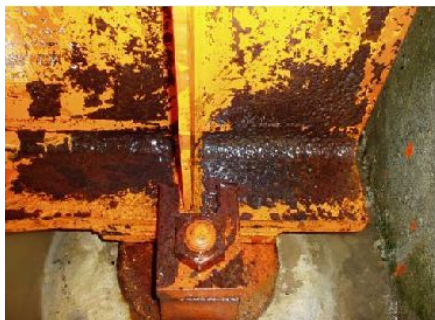
Fig.2-12 Cleaned steel plate by jet water
