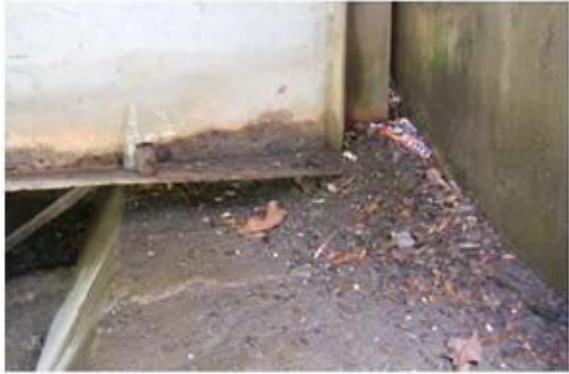
Photo 1-1-6 Debris on bearing
