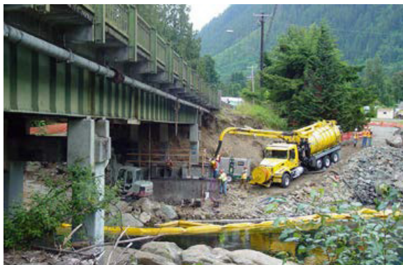
Figure 4-12 Scour repair work by special heavy equipment
