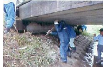
Fig.2-20 Mowing and Weeding under the bridge
