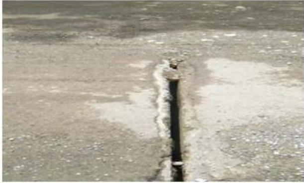
Photo 1-1-6 Debris on bearing
