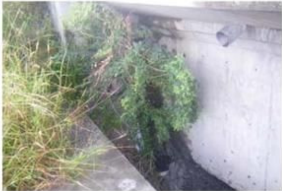
Photo 1-1-7 Vegetation on substructure
