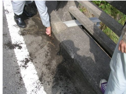
Fig.2-4 Removing the soil by brush
