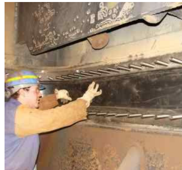
Fig.2-8 Cleaned expansion joint tube
