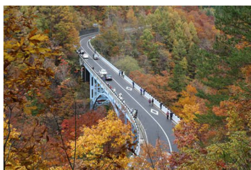
Fig.2-19 Tree growth under the bridge
