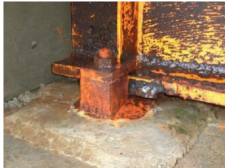
Fig.2-11 Cleaned Bearing by jet water
