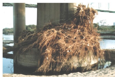
Caisson foundation Largely exposure of bottom plate surface
