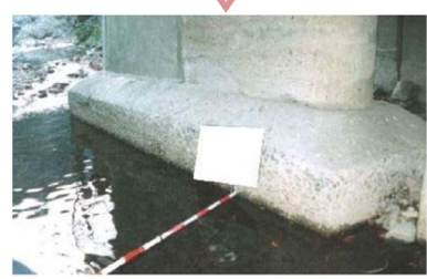
Spread foundation Exposure of the footing underside
