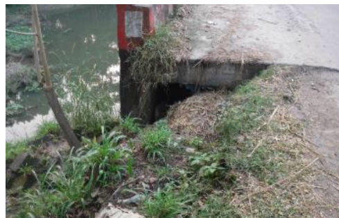
Collapses of embankments at the abutment
