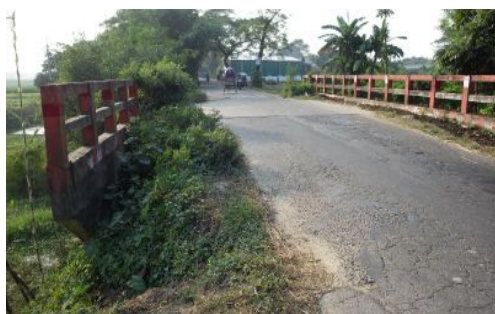
Collapses of embankments at the abutment
