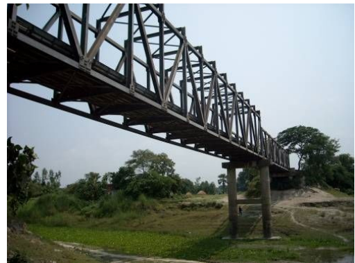
Rodal Tiki Portable Steel Bridge in Manikganj
