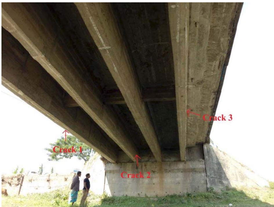
Photo 2-4 Position of Crack-1 to Crack-3
