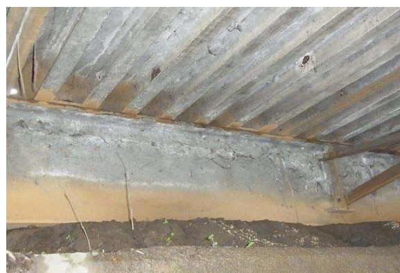
Photo 4 Accumulated debris around bearings
