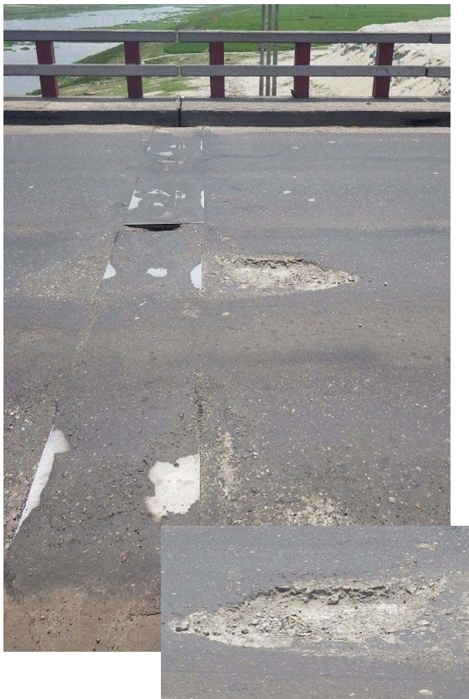
Photo 5: Pothole near expansion joint
