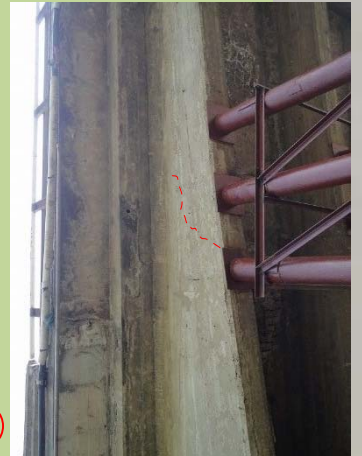
5 G3 : Cracks of Main Girder
