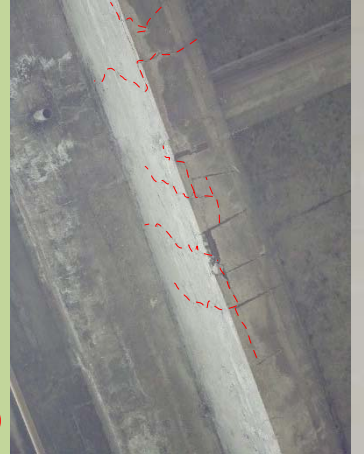
9 G1 : Cracks of Main Girder
