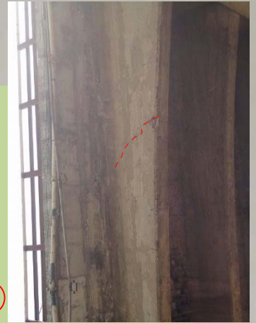
6 G3 : Cracks of Main Girder
