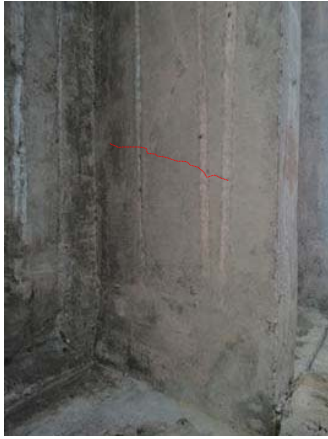
Photo No.2 P2-A2 G3 : Shear Cracks of main Girder
