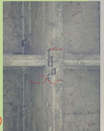
10 G2 : Cracks of Main Girder
