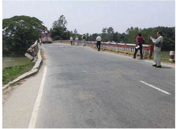
Photo 2 Bridge Surface, damaged RCC railing
