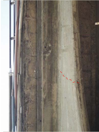
2 G1 : Cracks of Main Girder
