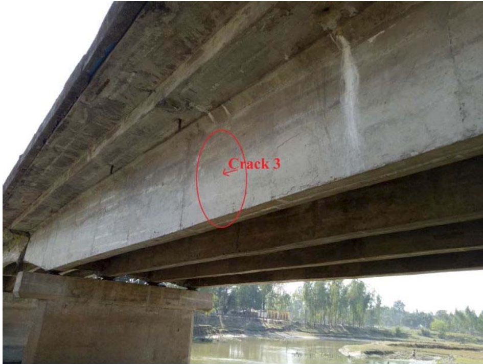
Photo 2-3 Position of Crack-3
