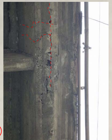
11 G3 : Cracks of Main Girder
