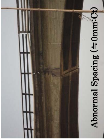
B P2-P3 : Gerber Type hinge
