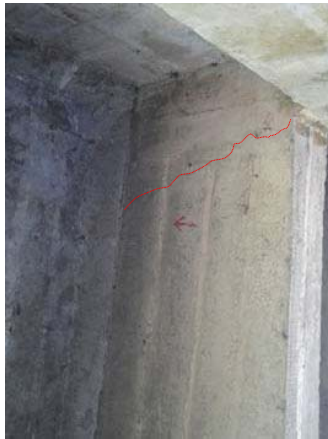
Photo No.3 A1-P1 G3 : Shear Cracks of main Girder
