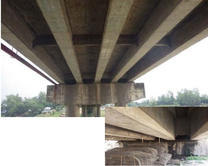
Photo 9: Underside of the Bridge (PC portion)
