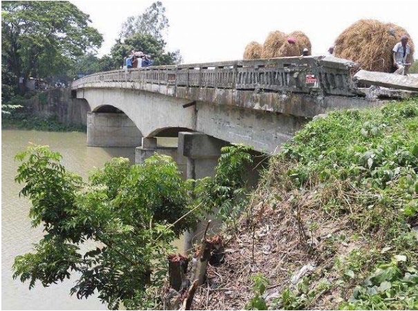
Photo 1 Side view, additional pier under Gerber-hinge
