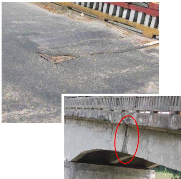
Photo 5 Damaged expansion joint above Gerber-hinge
