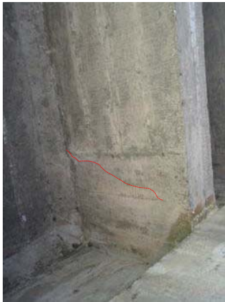
Photo No.3 A1-P1 G3 : Shear Cracks of main Girder
