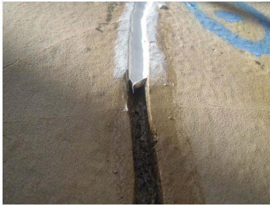
Photo 9 crack Filling
