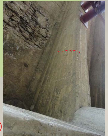
3 G2 : Cracks of Main Girder
