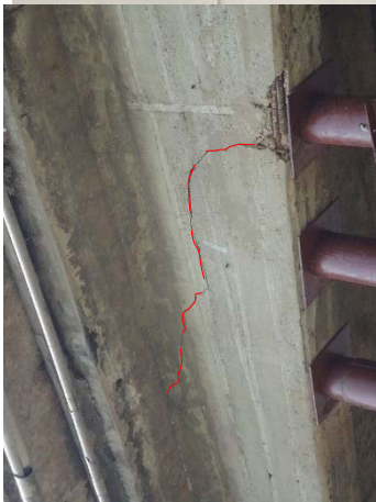
1 G1 : Cracks of Main Girder
