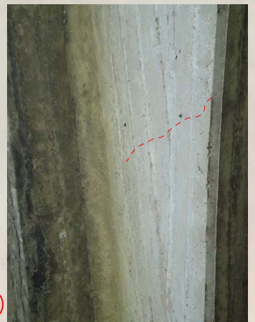
7 G3 : Cracks of Main Girder
