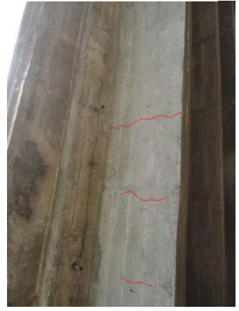
Photo No.4 A1-P1 G4 : Flexural Cracks of main Girder
