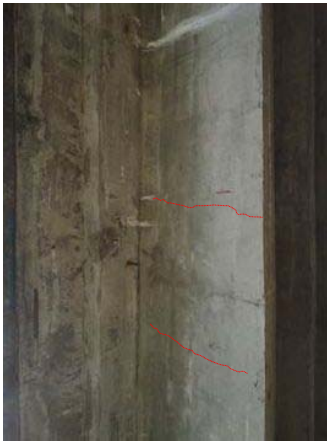
Photo No.5 A1-P1 G1 : Flexural Cracks of main Girder
