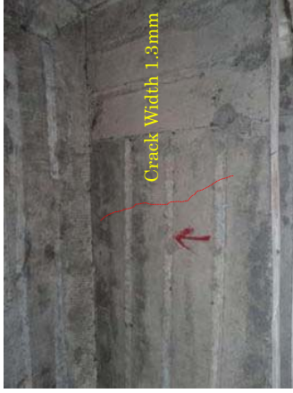
Photo No.2 P2-A2 G3 : Shear Cracks of main Girder
