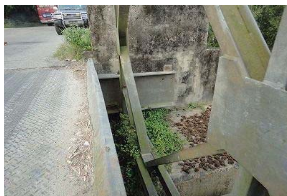
Photo 2 Unevenness and pavement crack of approach
