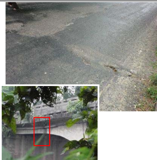
Photo 6 Buried expansin joint above Gerber-hinge
