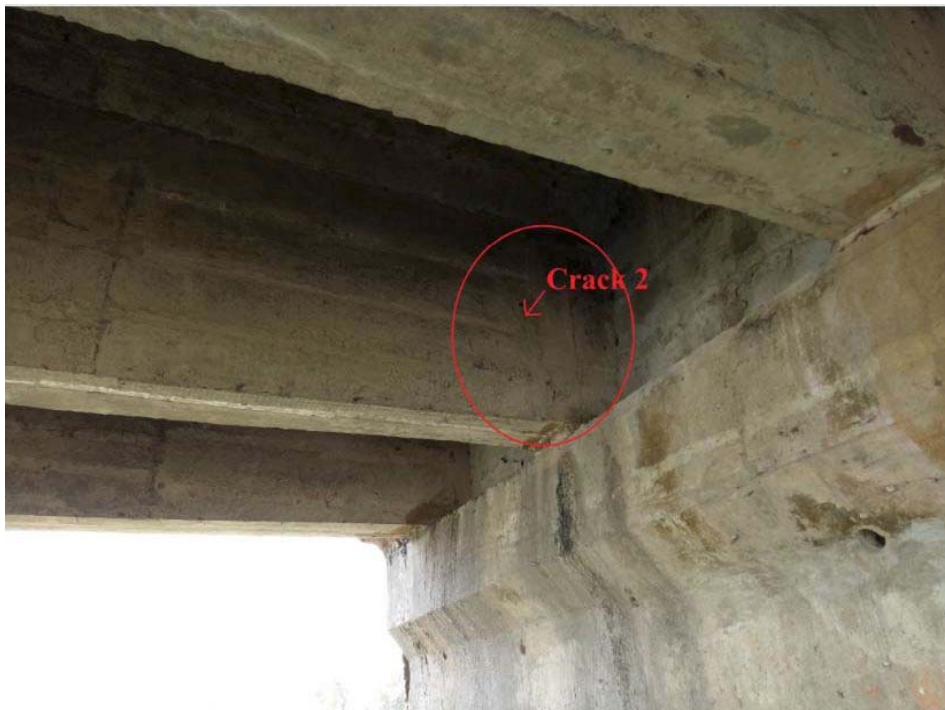
Photo 2-2 Position of Crack-2
