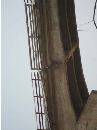
A P2-P3 : Gerber Type hinge
