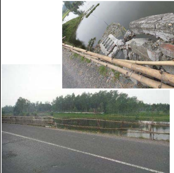
Photo 3 Missing of railing
