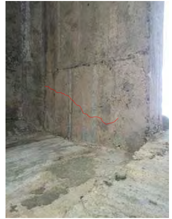
Photo No.1 P2-A2 G4 : Shear Cracks of main Girder
