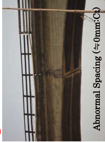
(B) P2-P3 : Gerber Type hinge
