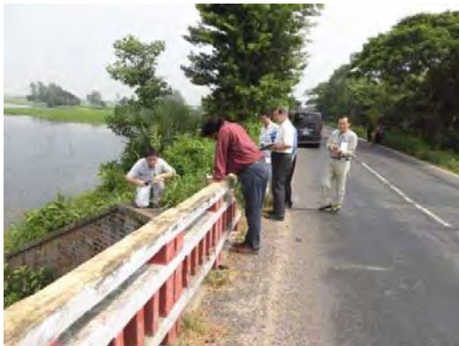
Site survey of brick abutment
