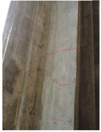
Photo No.4 AI-P1 G4 : Flexural Cracks of main Girder
