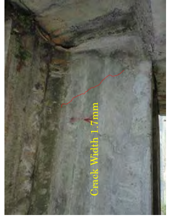
Photo No.1 P2-A2 G4 : Shear Cracks of main Girder
