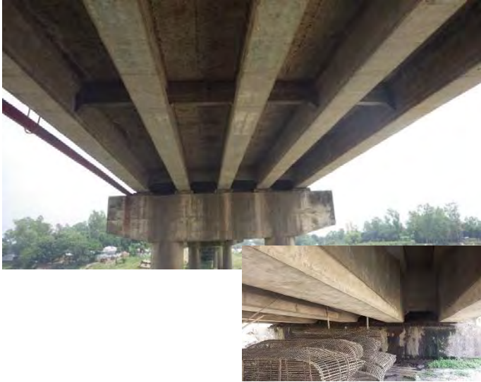
Photo 9: Underside of the Bridge (PC portion)
