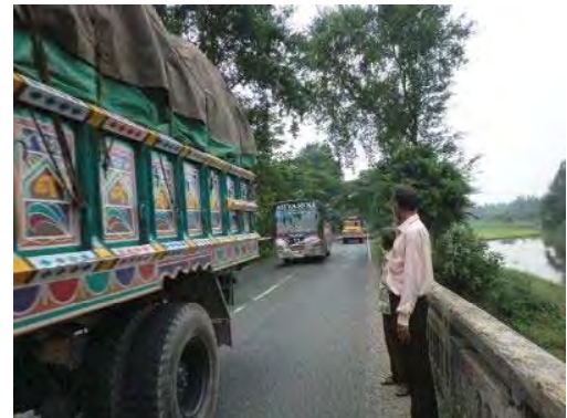
No side walk (Insufficient width of shoulder)
