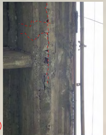
11 G3 : Cracks of Main Girder
