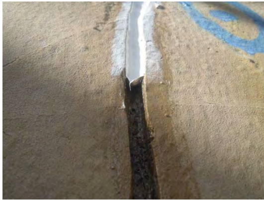
Photo 9 crack Filling
