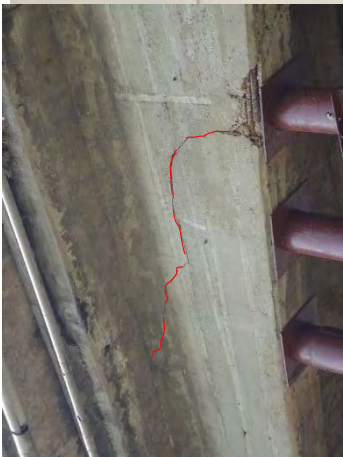
1 G1 : Cracks of Main Girder
