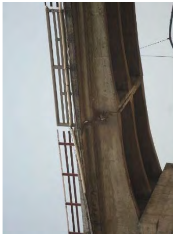
(A) P2-P3 : Gerber Type hinge
