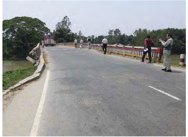
Photo 2 Bridge Surface, damaged RCC railing
