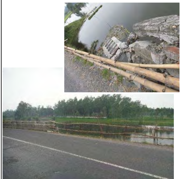
Photo 3 Missing of railing
