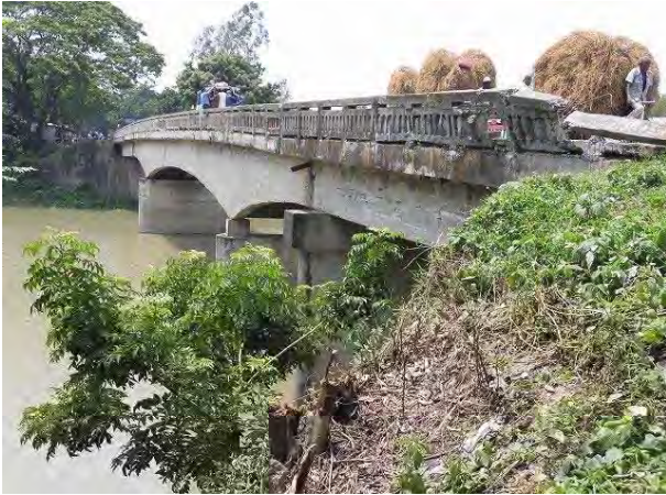
Photo 1 Side view, additional pier under Gerber-hinge
