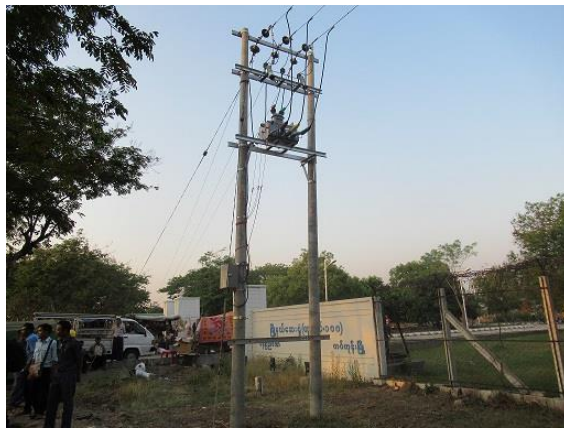
Figure 2-11: Switch Gear and Transformer Installed to the Actual Distribution Line (Left: Switch Gear in Tatkon, Right: 3-Phase Transformer in Tatkon)
