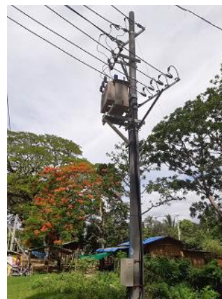
Figure 2-11: Switch Gear and Transformer Installed to the Actual Distribution Line (Left: Switch Gear in Tatkon, Right: 3-Phase Transformer in Tatkon)
