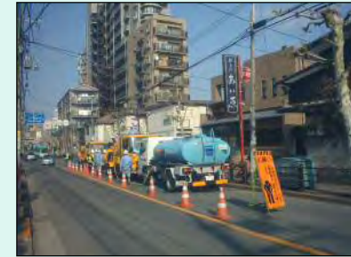
Overview of Cleaning Works Sites
