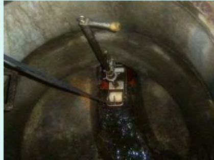
Setting up of Guide Roller to protect pipe
