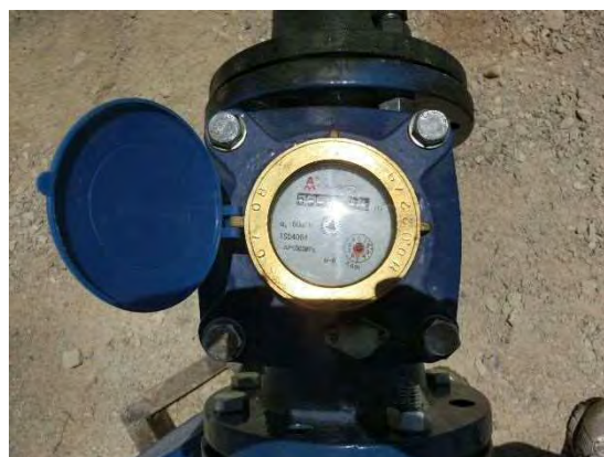
Photo-4 Bulk Meter for Irrigation
