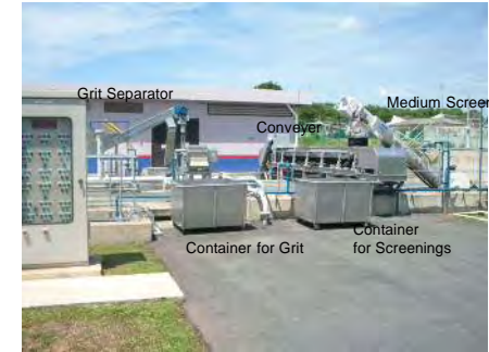
Grit Chamber (Image)
