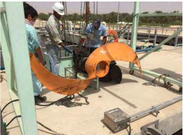
Trouble-shooting 1 Inspection of reactor mixer after lifting up
