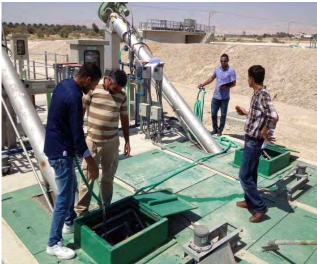
Cleaning work of fine screen at the grit chamber
