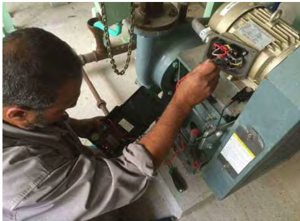
Trouble-shooting 2 Inspection for earth leakage of motor
