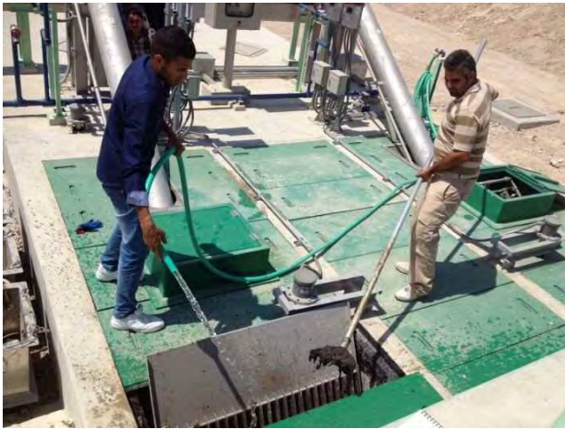
Removal of screenings at the coarse screen
