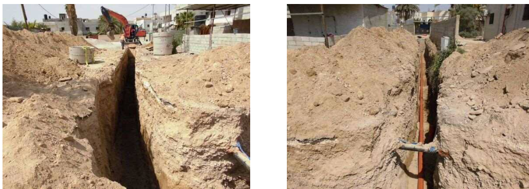
Figure 2.22.2 Sewer Construction in AJ Camp
