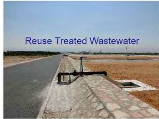
Irrigation tapping point for cleaning drying bed
