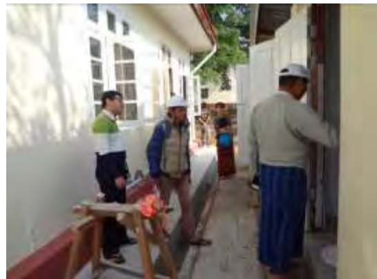
Monitoring the renovation process
