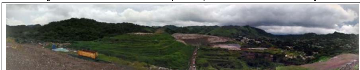
Figure 2.3.20 Phase 2 and 3 landfill sites viewed from Phase 1 site
