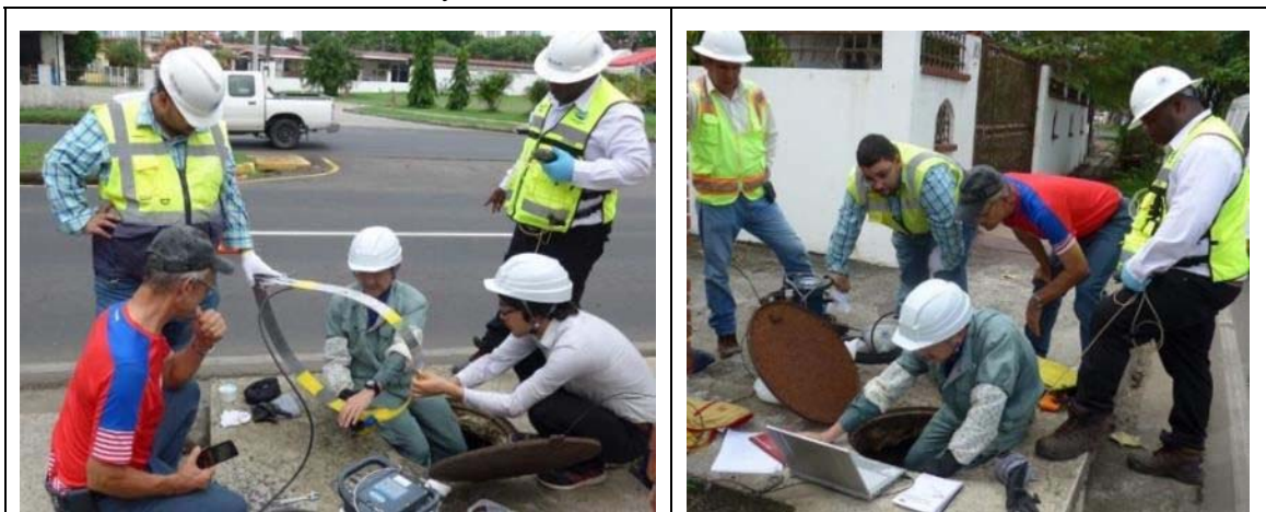
Figure 2.3.18 Installation of open channel flowmeter and data setting
