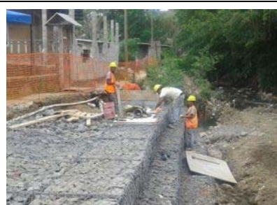
Fig. 2.3.8 Repairing the collector
