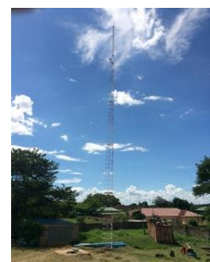
Existing Antenna Tower
