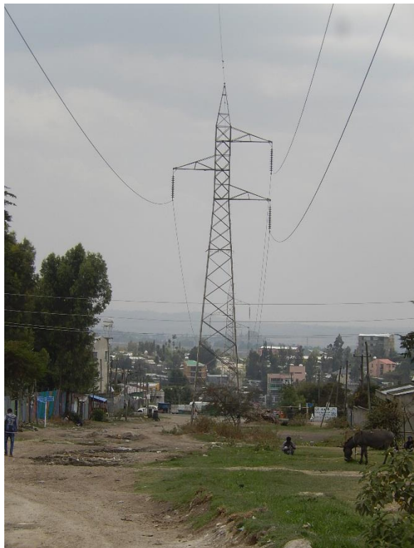
T 28 DSCN0561 T28 from T27 side
