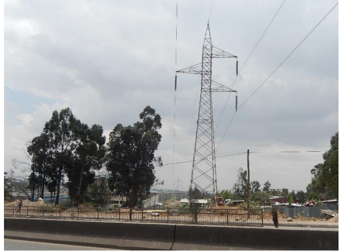
T34 DSCN0494 T34 Elevation level of road is 5 meter higher than elevation of T34. Electrical clearance to road is not enough.
