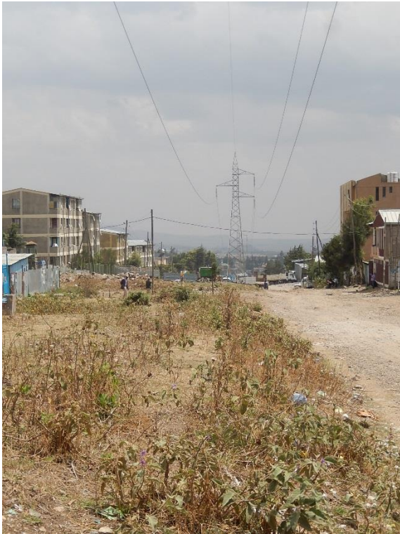
T 27 DSCN0572 T27 from T26 side
