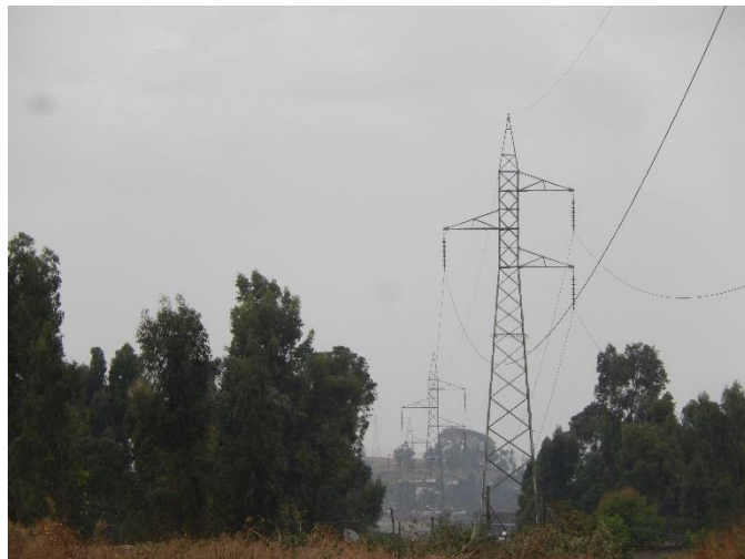
T43 DSCN0788 T43 from T42 Along the fence for water treatment, many houses are constructed. ROW (Corridor is disappeared).
