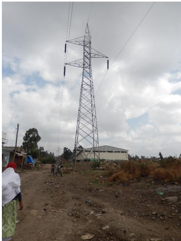
T 35 DSCN0708 T35 from T 36 side.
