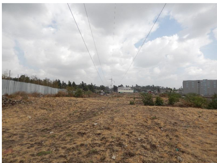
T 35 DSCN0715 T35 from T36 side. Surrounding area of ROW (Corridor) become a part of industrial area, The elevation of the arear has been level up by embankment works.
