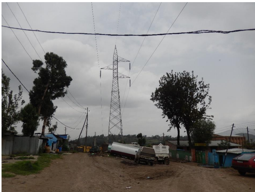
T20 on the slope toward existing road.
