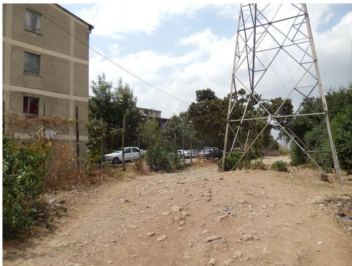
T 25 DSCN0592 T25 near existing road and fence
