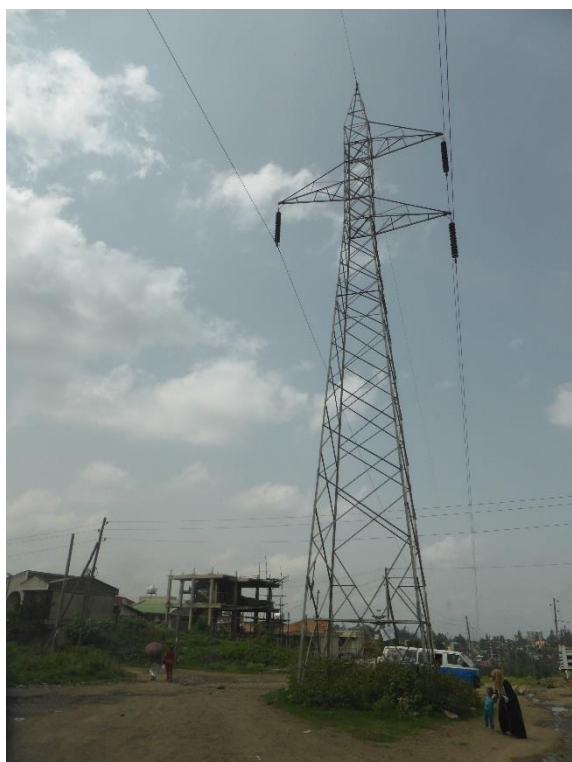
T 29 DSCN0561 T28 from T28 side
