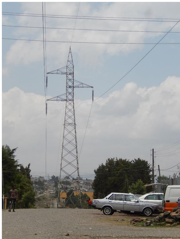
T 32 DSCN0511 T32 from T33 side
