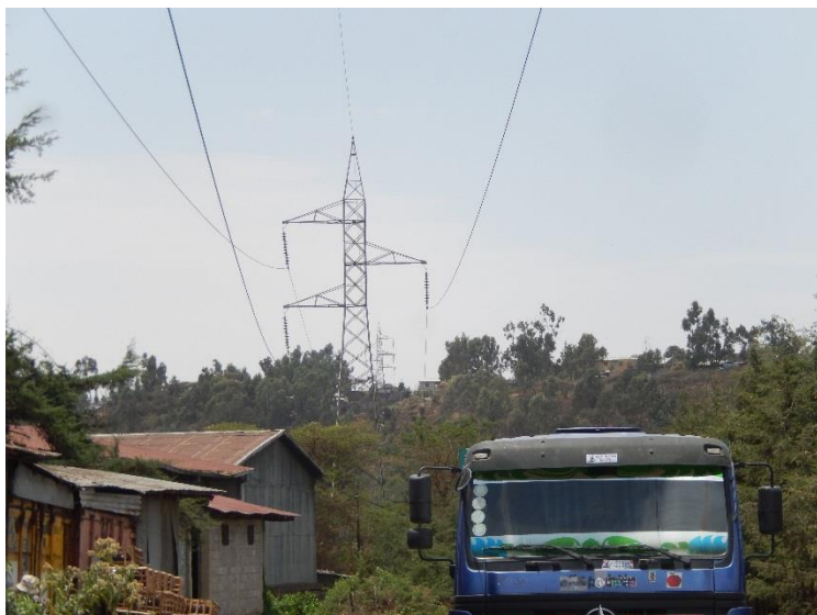
T 22 DSCN0983 T22 view from T21 : Transposition.
