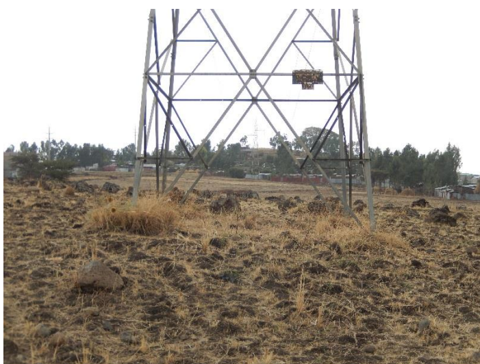
DSCN0833 T50 bottom Residential houses are existed toward T51.
