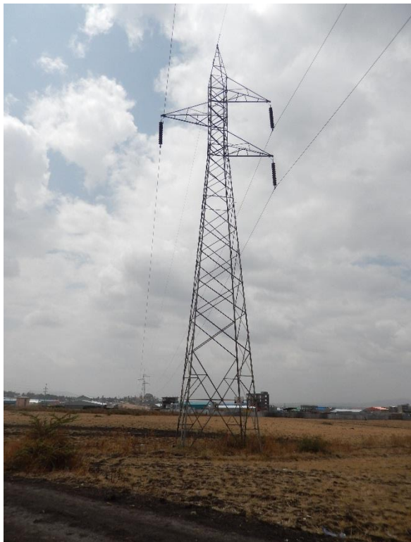
T 45 DSCN0801 T45 from T 44 side
