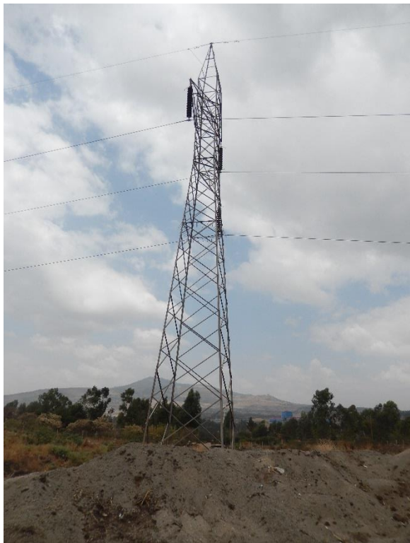
T 42 DSCN0783 T42. Embankment works were done around tower site/
