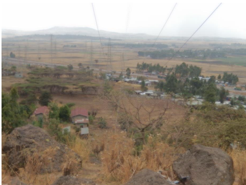
DSCN0844 View from T 52 toward T53 and T55 where are inside the Kaliti-I substation.
