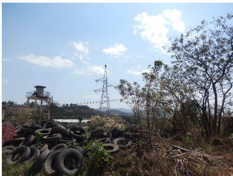
Dead-end Tower toward Mekanissa substation DSCN0273 DE Tower
