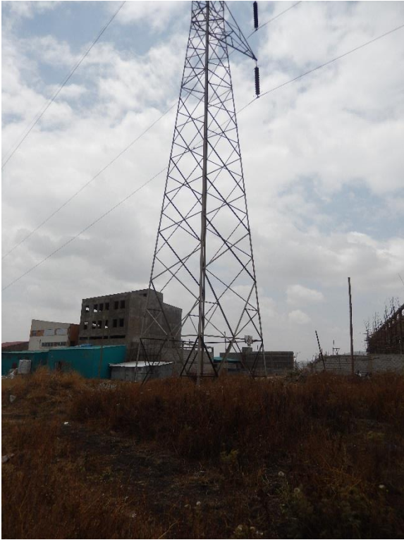
T 47 DSCN0812 T47 from T46 side.
