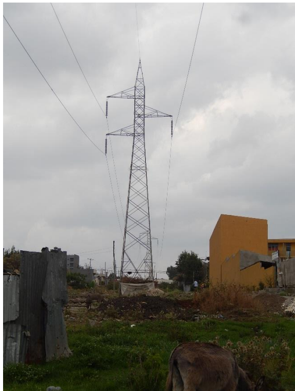
T 30 DSCN0540 T30 from T 29 side
