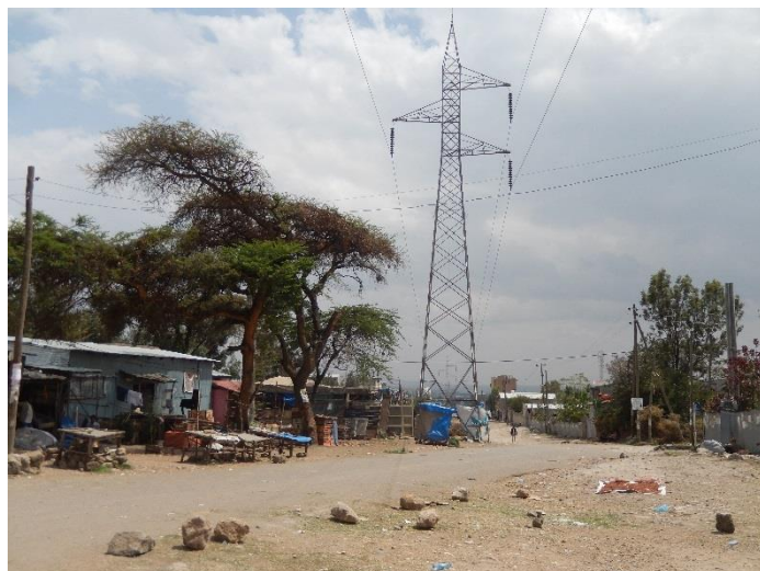
T 26 DSCN0582 T26 from T25 side showing Tree & ROW
