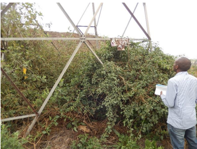
T 40 DSCN0761 T40 Bottom Embankment
