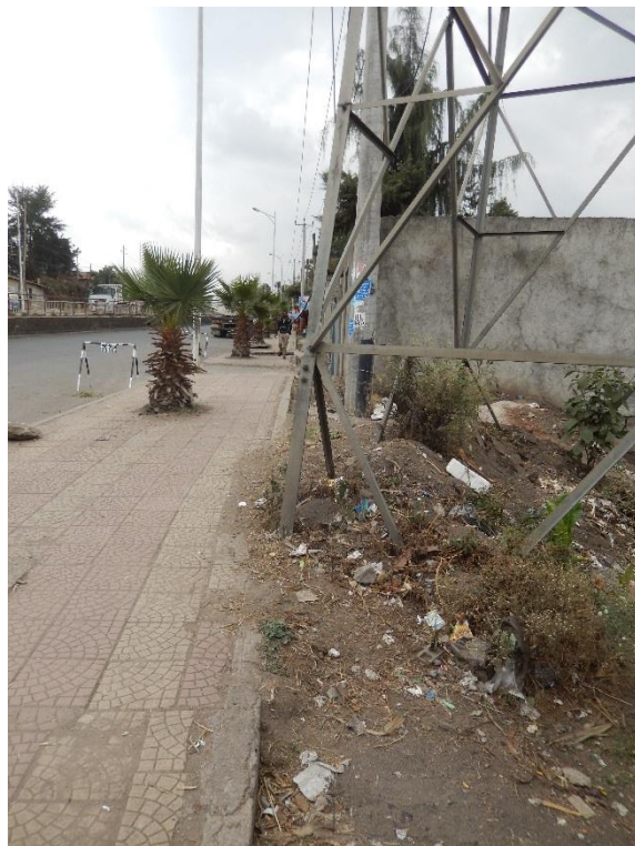
T 31 DSCN0529 T31 Tower Legs are located in road edges.
