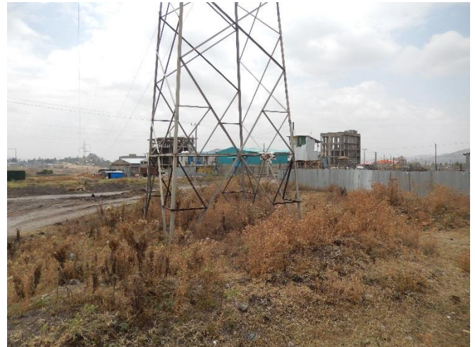
T46 DSCN0809 A view from T 46 toward T47. ROW (Corridor) is maintained. New factories are constructed out side the ROW.
