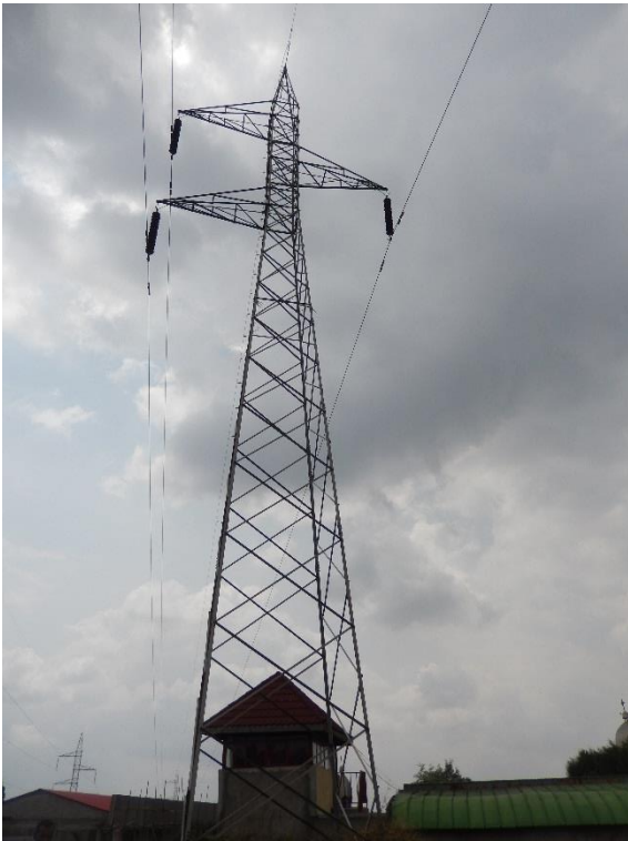
T 67 DSCN0387 New T-Branch to Weregenu Substation
