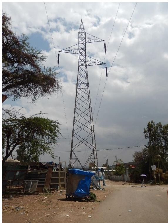
T 26 DSCN0579 T26 from T25 side
