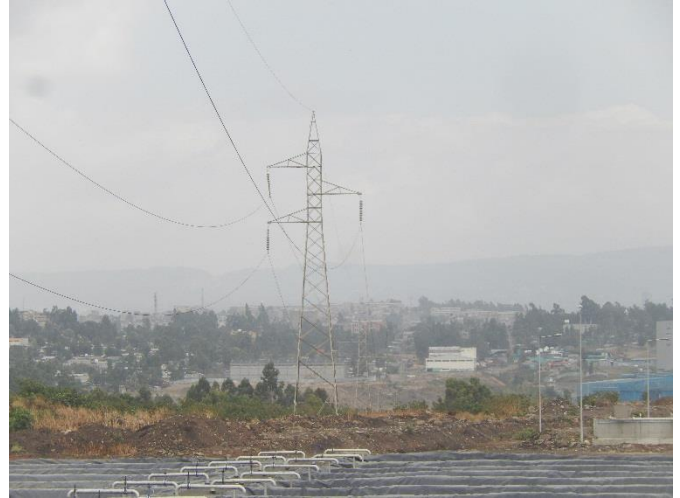
T41 DSCN0785 T41 from T42 side. Transmission line pass the area of water treatment. An access road is belonging to water treatment. ROW (Corridor) is not so clear, but no houses.
