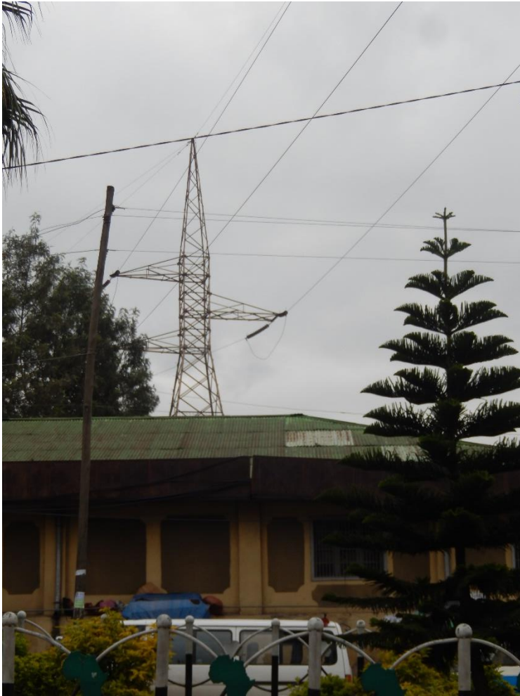
T-01 views from Main Road. T-01 is dead-end tower to Addis Center Substation
