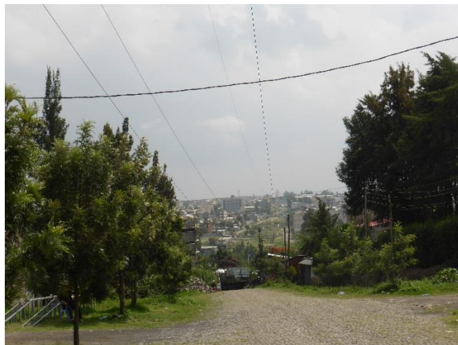
ROW (Corridor) between T 31 and T32 P1130596 T32 view toward T31, many residential houses are existing.
