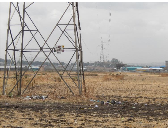
T 44 DSCN0799 T44 from T43 side
