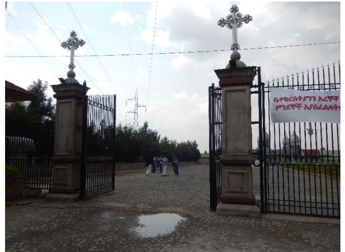
T 67 DSCN0367 New Tower will be located 30-40 meter front of existing tower T67.
