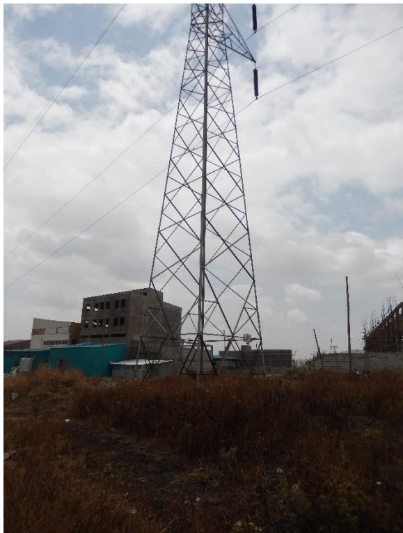
T 47 DSCN0812 T47 from T46 side.
