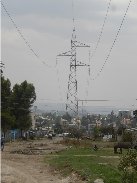
T 28 DSCN0561 T28 from T27 side
