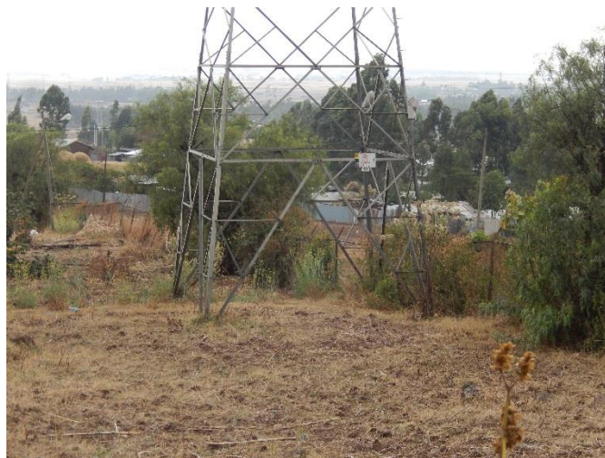
T 52 DSCN0851 T53 is located inside Kaliti-I substation.
