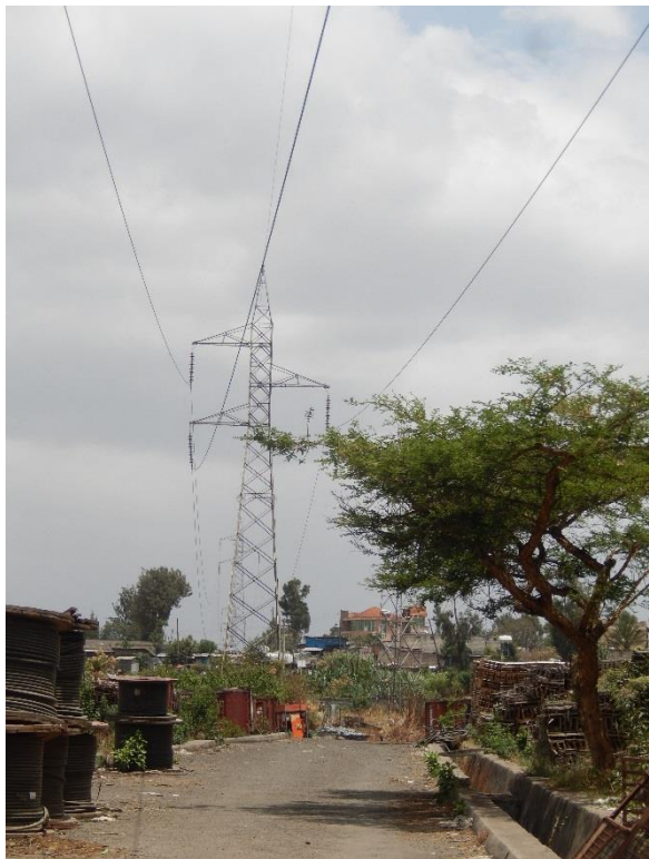
T 21 DSCN0982 T21 view from T22 side Transposition Tower
