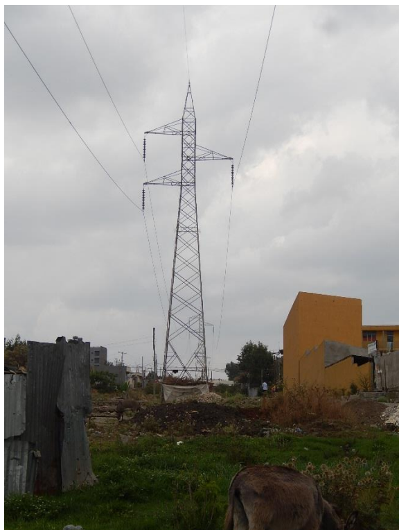
T 30 DSCN0540 T30 from T 29 side
