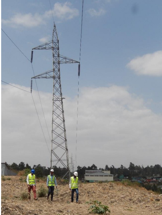
T 36 DSCN0906 T36 from T37 side.
