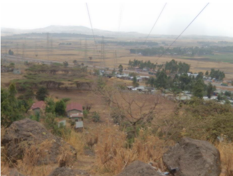
DSCN0844 View from T 52 toward T53 and T55 where are inside the Kaliti-I substation.
