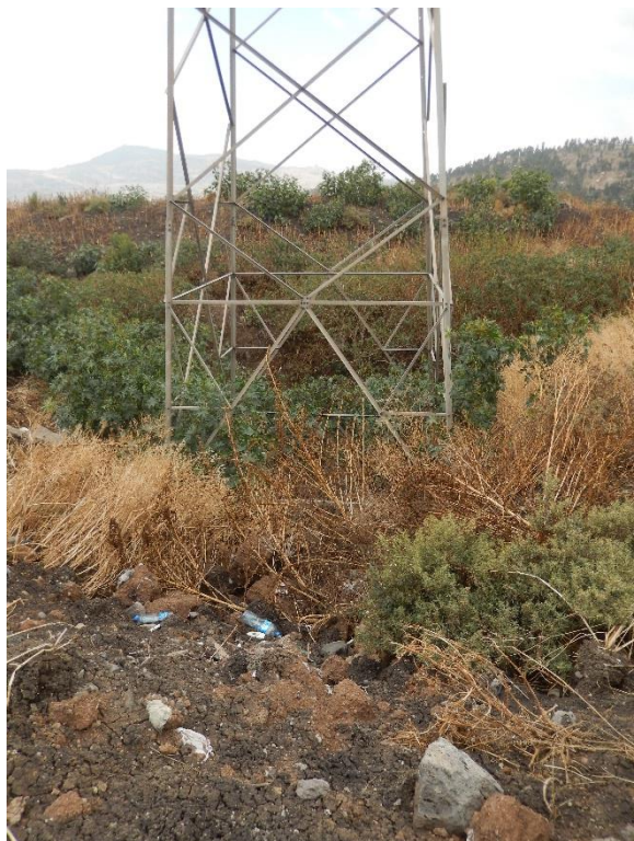
T 40 DSCN0773 T41 foundation. Embankment works were done around tower site/
