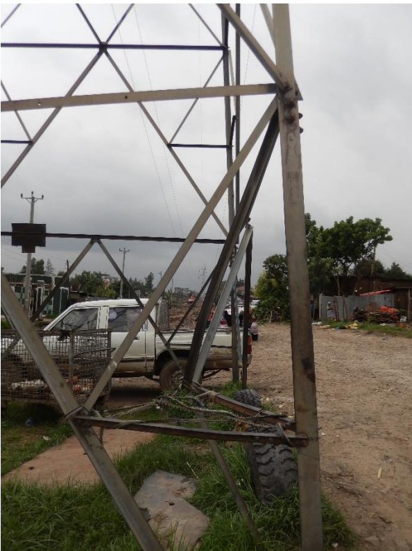
T18 Damaged Leg steels
