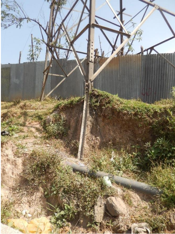
T52 Kaliti – Sebeta Existing Foundation No concrete Chimney for stub DSCN2408
