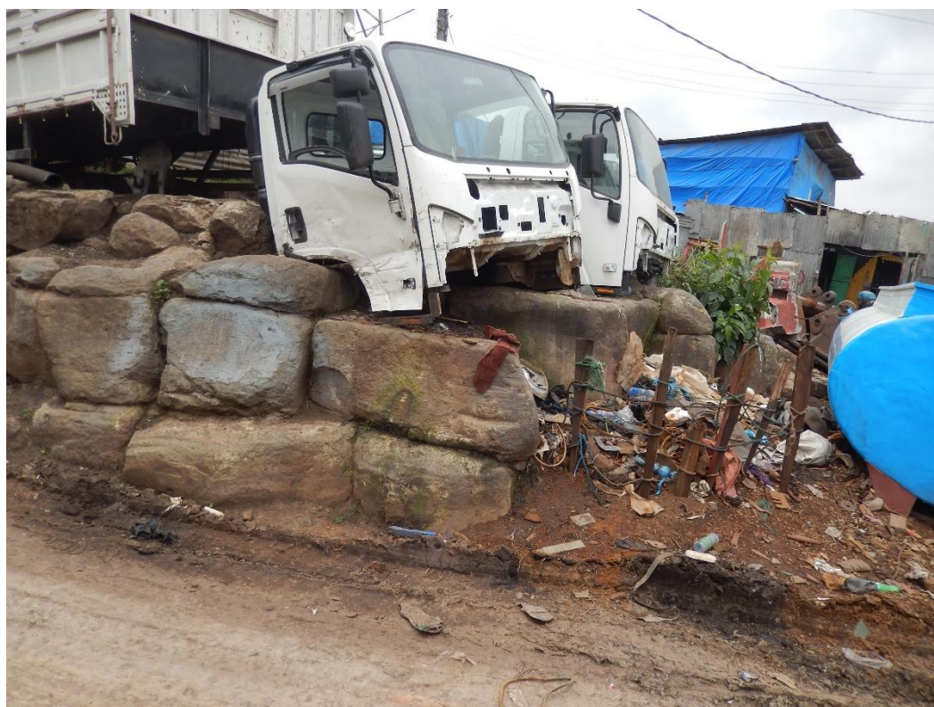
T20 on the slope toward existing road. Here will be end of new construction road
