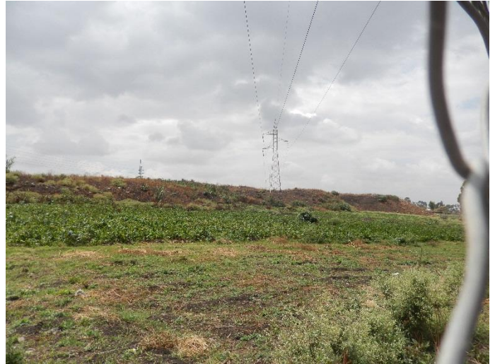
T40 DSCN0772 T40 from T39 side. Tower is located inside the water treatment area with boundary fence.
