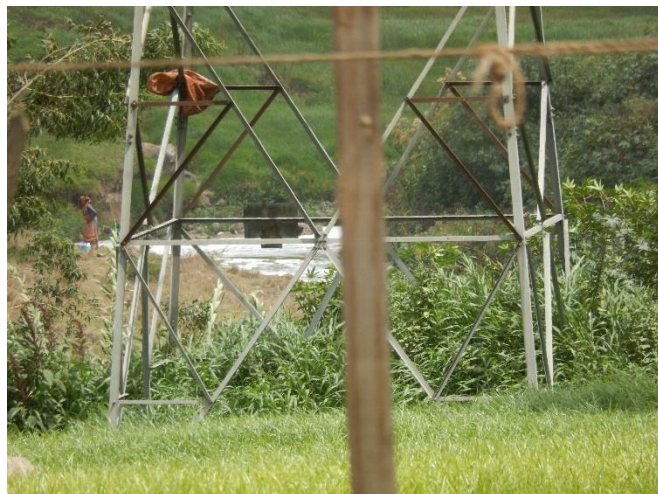
T39 DSCN0770 T39 & river. Access bridge to cross river is for light weight only. Vehicle is not accepted to cross.
