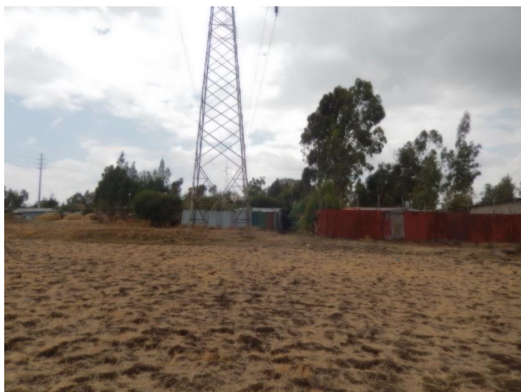
DSCN0838 T51 bottom Residential houses are existed between T51 to T52.
