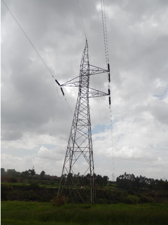
T 38 DSCN0744 T38 from T37 side. Tension tower with OPGW Joint Box. The deviation angle is small.
