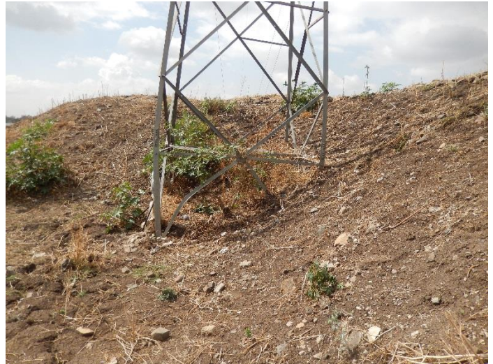
T36 DSCN0717 T36 Bottom Main leg was damaged and bent by soil pressures or hit by heavy equipment.
