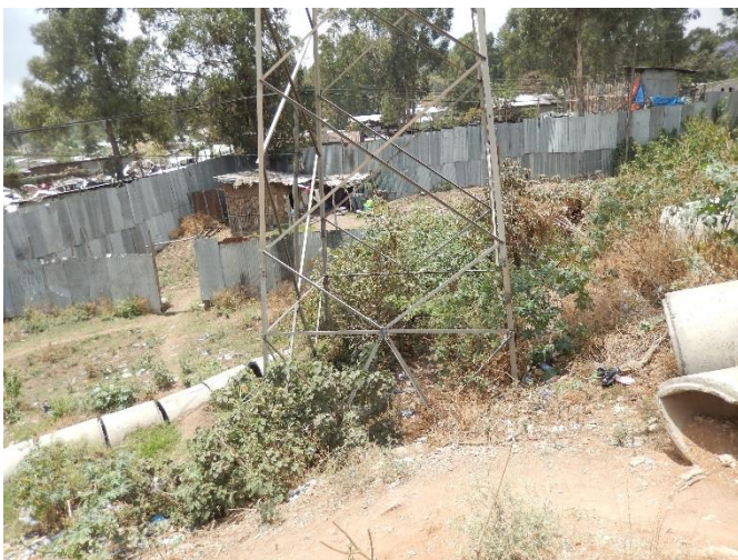
T 34 DSCN0485 T34 beside road. Water drain pipes for road are installed beside tower foundation.
