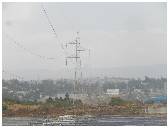
T41 DSCN0785 T41 from T42 side. Transmission line pass the area of water treatment. An access road is belonging to water treatment. ROW (Corridor) is not so clear, but no houses.
