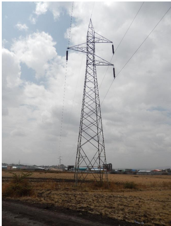
T 45 DSCN0801 T45 from T 44 side
