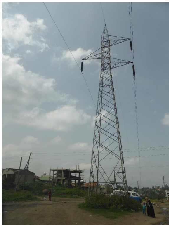
T 29 DSCN0561 T28 from T28 side
