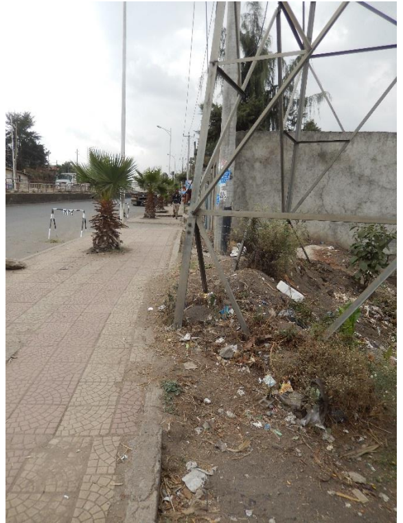
T 31 DSCN0529 T31 Tower Legs are located in road edges.
