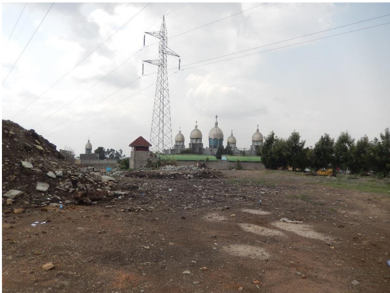
DSCN0379 T67 Second 132kV TL is just beside T67.
