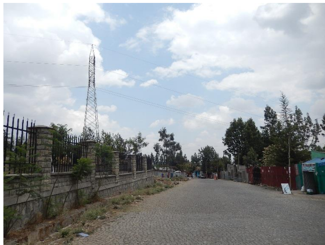
T33 DSCN0499 T33 from side 100m. Heavy weight span due to ground profile level toward T34.
