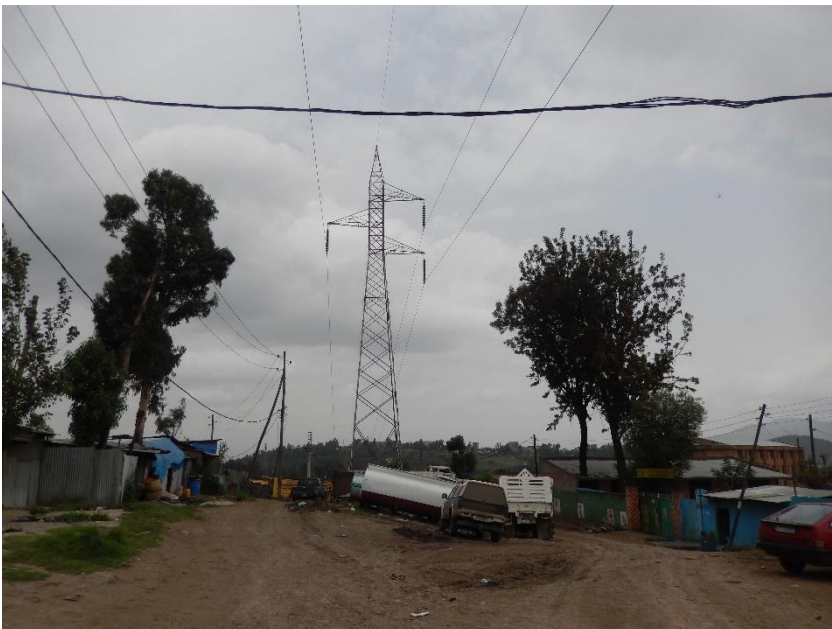
T20 on the slope toward existing road.
