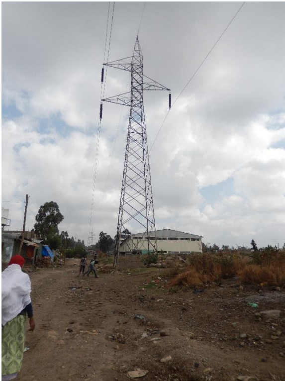
T 35 DSCN0708 T35 from T 36 side.
