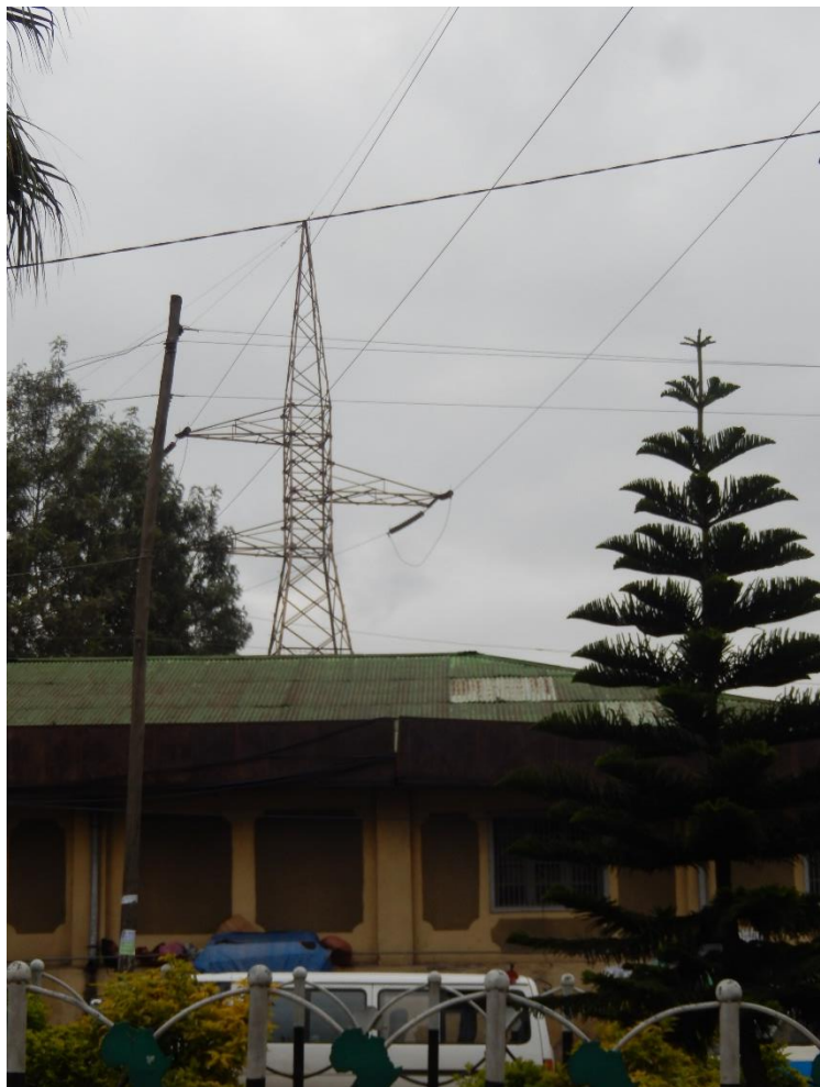
T-01 views from Main Road. T-01 is dead-end tower to Addis Center Substation
