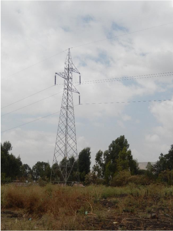
T 43 DSCN0791 T43 side residential houses. Hoses are constructed under ROW (Corridor) after T 42 water treatment area.
