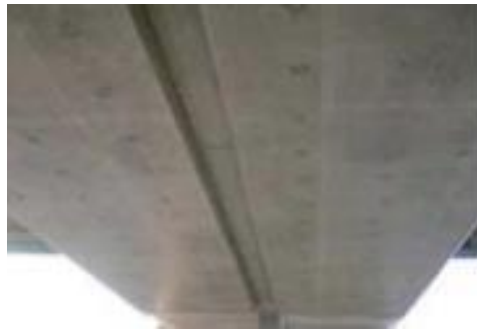
Figure 4 Application of "Skeleton Disaster Prevention Coating"
