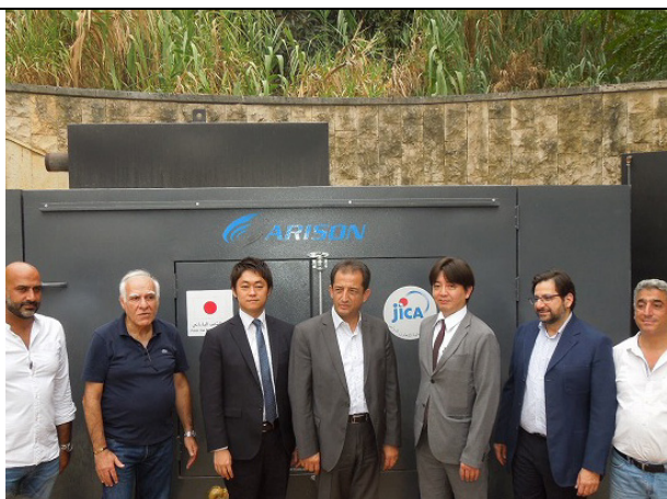
The generator installed at the water facility in Choueifat municipality.
