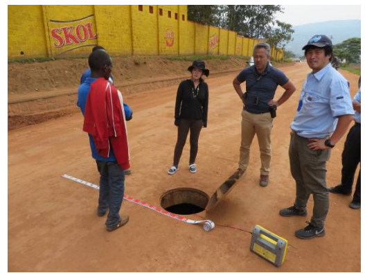
Site visit (Existing pipeline)
