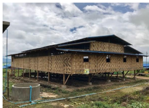
Figure 5.4.4 Layer Chicken Housing (Shan Highland Livestock Zone 1)
