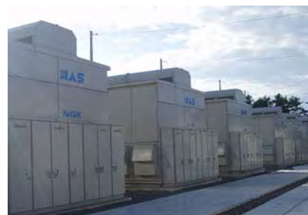
Sodium sulfur battery (34MWh system)
