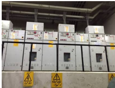
Figure 2-8-1-10 Low Voltage Switch Gear for chillers and BMS
