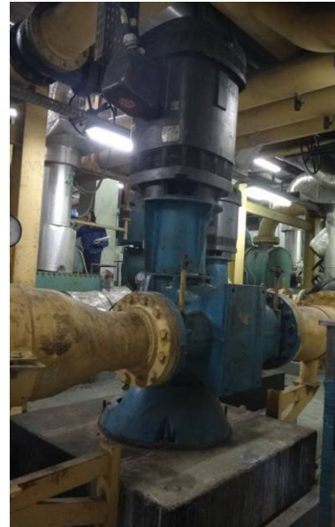
Figure 2-8-1-11 Chillers and condenser water pumps
