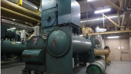
Figure 2-8-1-11 Chillers and condenser water pumps
