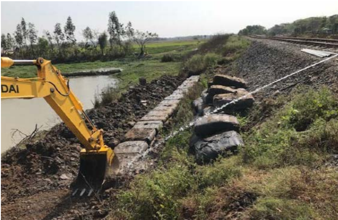
Image- 3 Countermeasure against the Slope Failure (by D • Box Dam Method)
