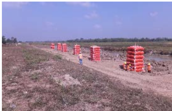
Image-5 Measurement of the Consolidation Subsidence (The original ground was good quality ground. Thus, D • Box's positive effect against the consolidation subsidence was not verified as a result of the one year measurement.)
