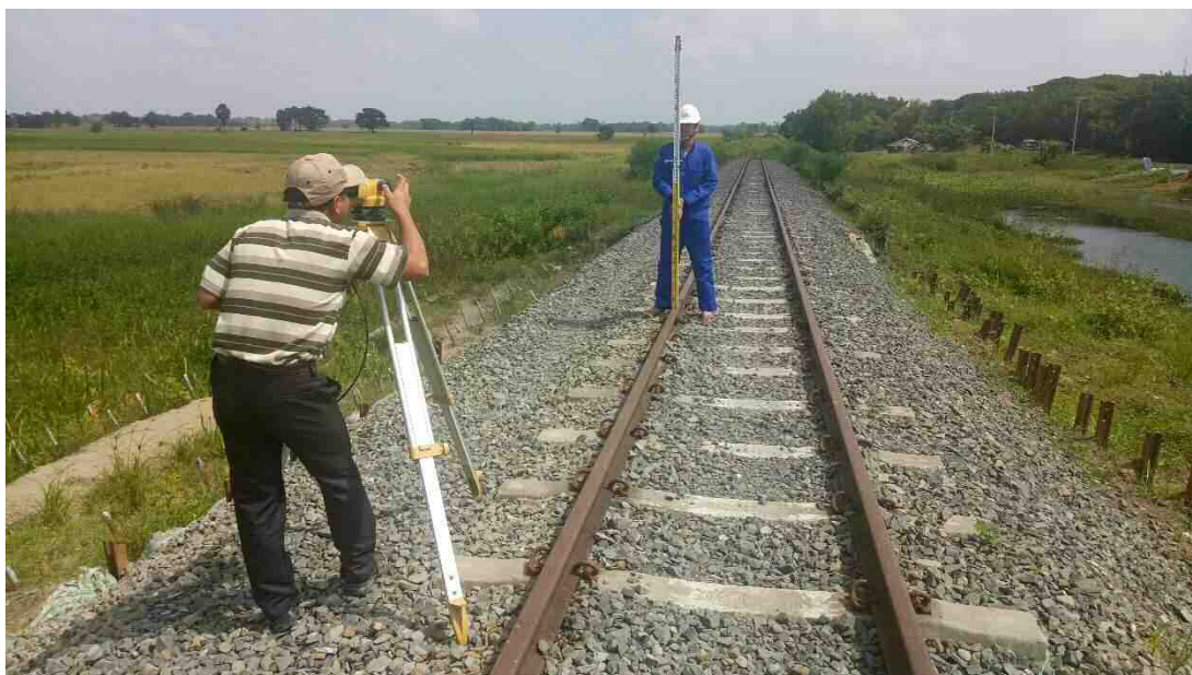
Photo - 2.1 Measurement Condition of Settlement of Railway Truck
