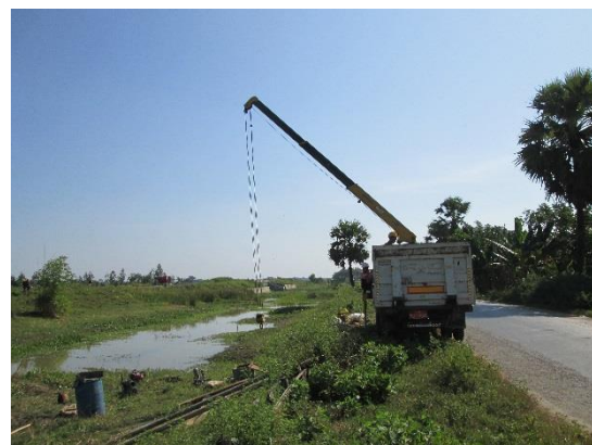
Photo - 1.6 Demobilization of Equipment
