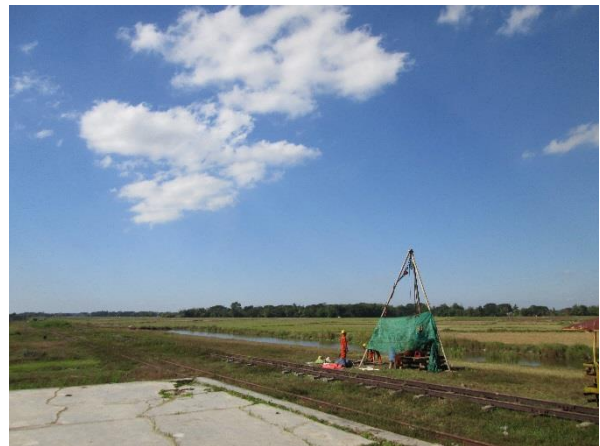
Photo - 3.2 View of BH-02
