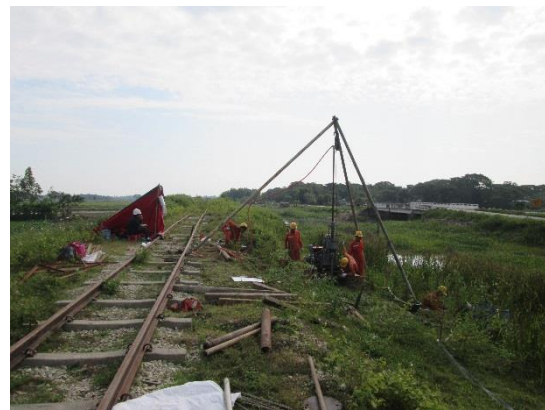
Photo - 1.4 One of drilling condition
