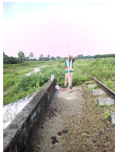
Photo - 3.6 TBM-2 (Panoramic View)
