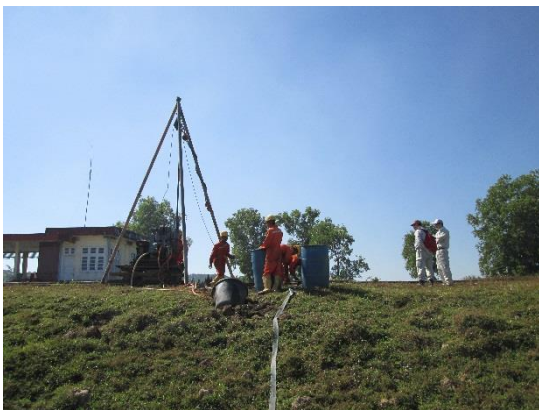
Photo - 1.3 One of drilling condition
