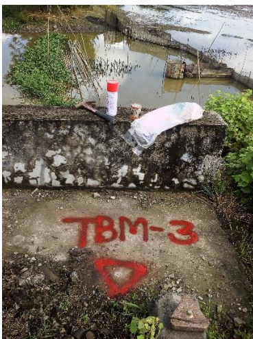
Photo - 3.7 TBM-3 (Panoramic View)
